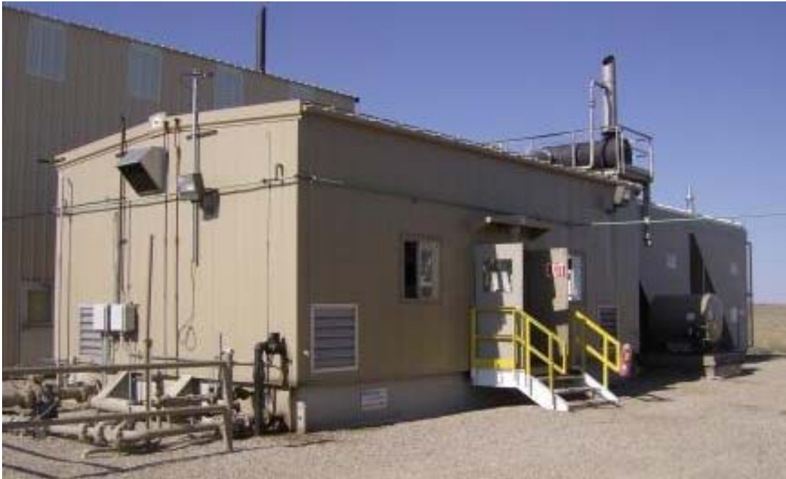
Figure 5: Compressor station external view, with engine room (in foreground) and exhaust stack/tailpipe on elevated catwalk (in background)
