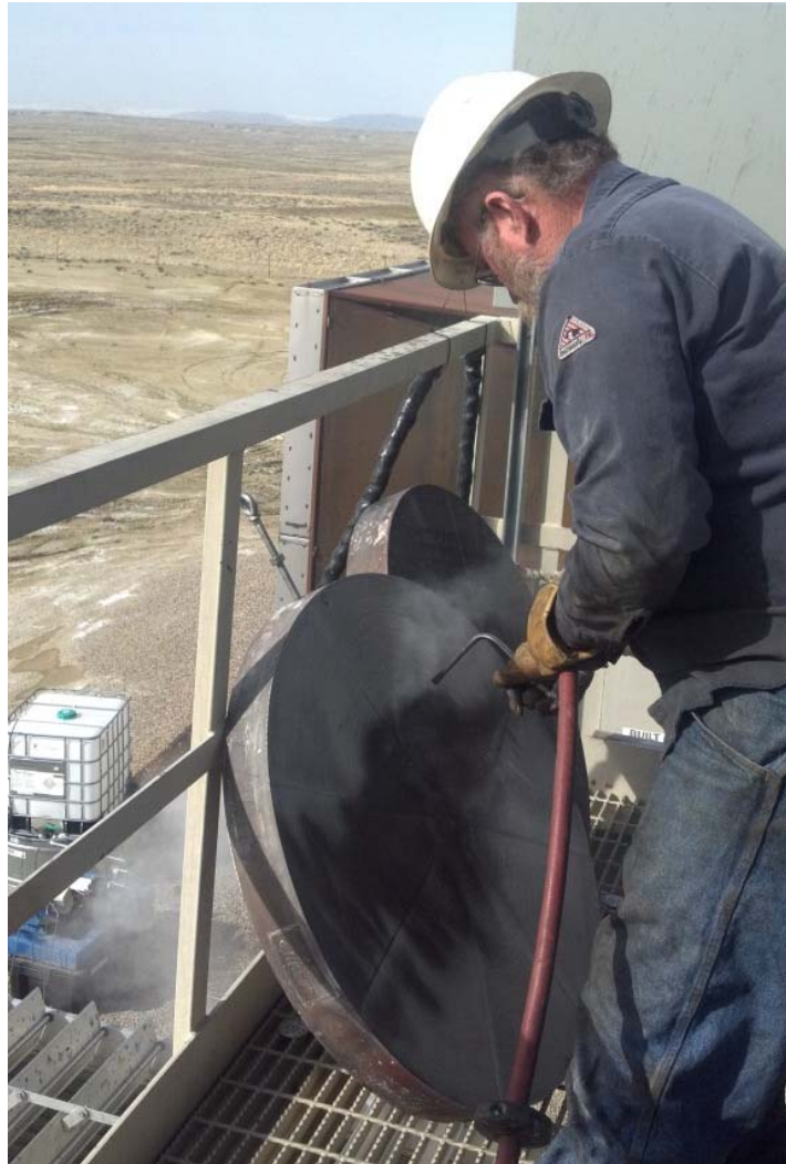
Figure 26: Catalyst elements being blown out with compressed air to clear ash-masking.
