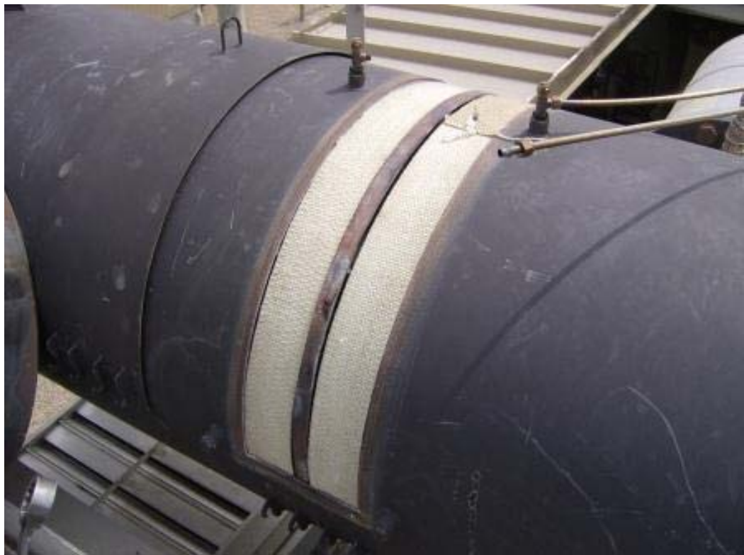
Figure 10: Emit elements in the catalyst housing (leading element is on the right), with thermal-wrap around the frame for proper sealing. Direction of exhaust gas flow is from right to left.
