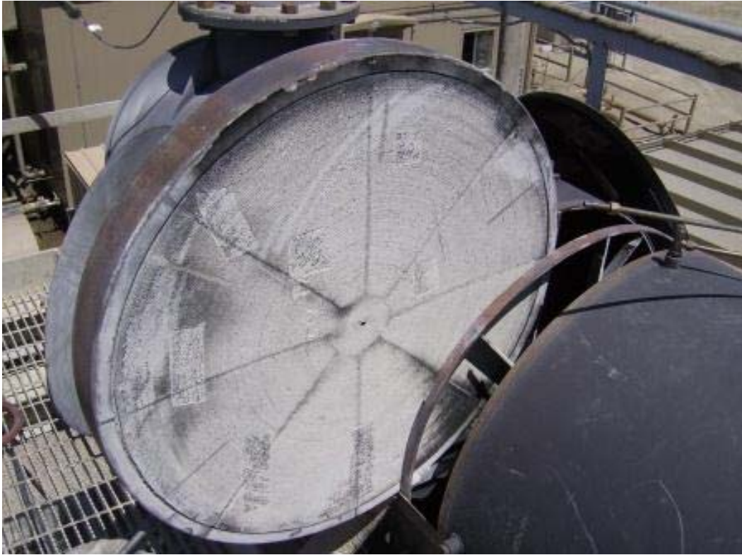
Figure 9: Lagging catalyst element (with ash on front face) being removed from the housing for cleaning.
