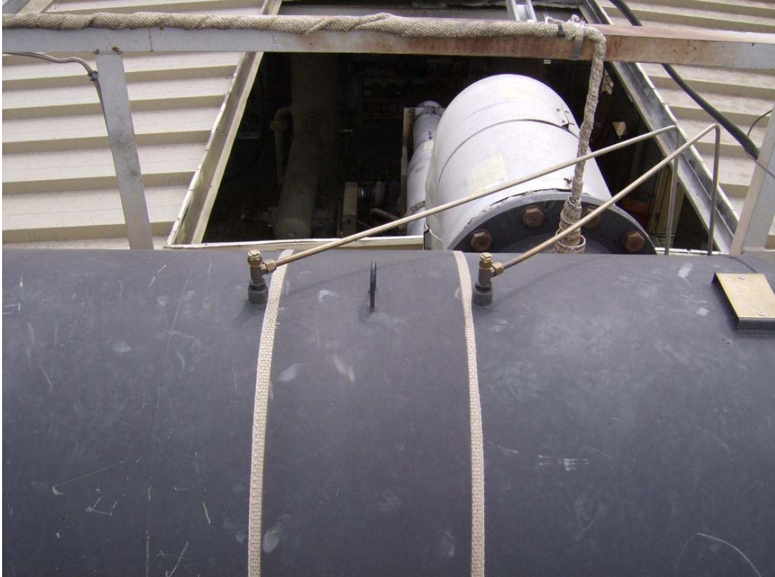
Figure 28: Pre (right) and post (left) catalyst pressure taps affixed atop the catalyst housing.
