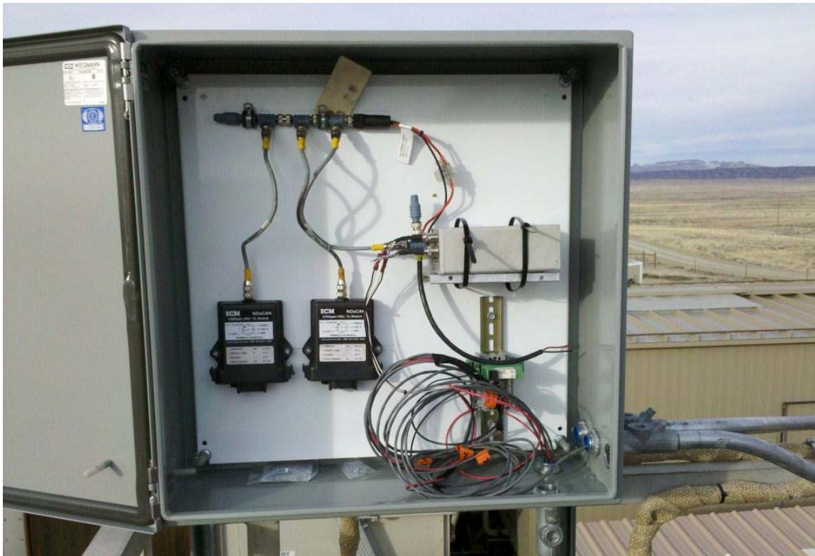
Figure 22: NOx sensor control module installed inside sealed enclosure on elevated catwalk.
