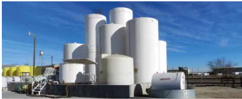
Liquid fertilizer storage facility
