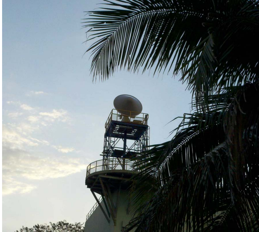
Figure 1.1: CSU-X25P radar node mounted atop R&D Center, UPRM campus
