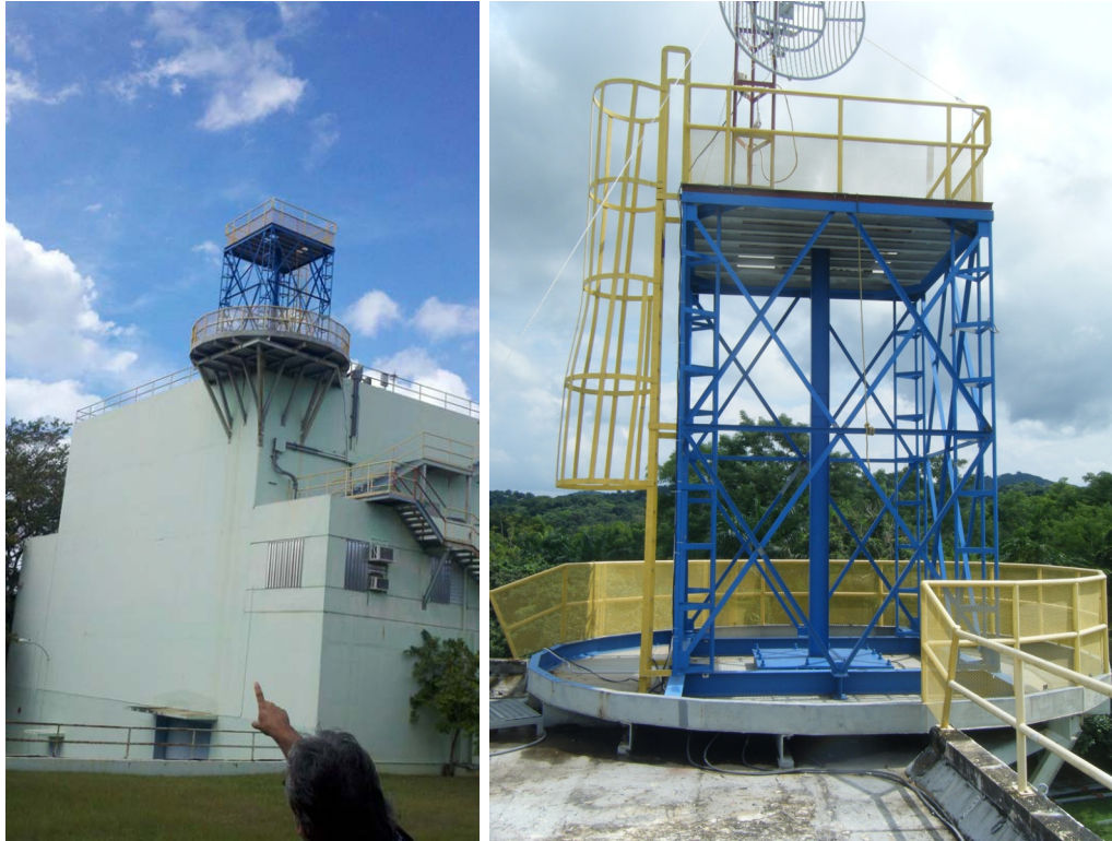
(a) Tower on R&D Building
