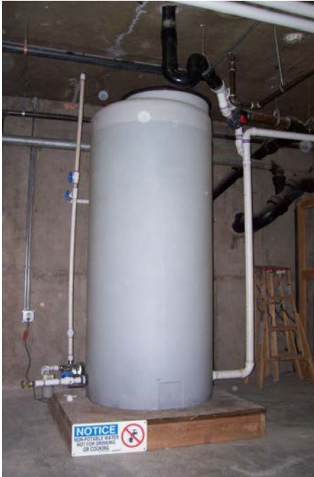
Figure 4.4 Graywater Collection Units Located in the Basement of the Residence Halls. (Right) shows 300 gallon tank in Edwards Dorm. (Left) shows a 300 gallon collection tank located in Aspen Hall.
