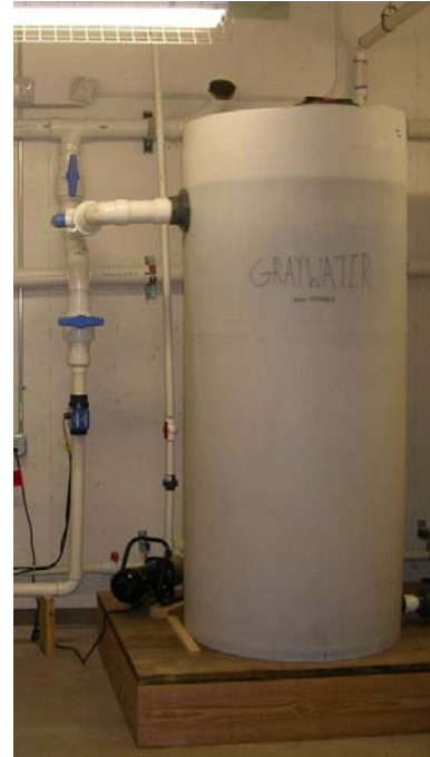
Figure 4.4 Graywater Collection Units Located in the Basement of the Residence Halls. (Right) shows 300 gallon tank in Edwards Dorm. (Left) shows a 300 gallon collection tank located in Aspen Hall.
