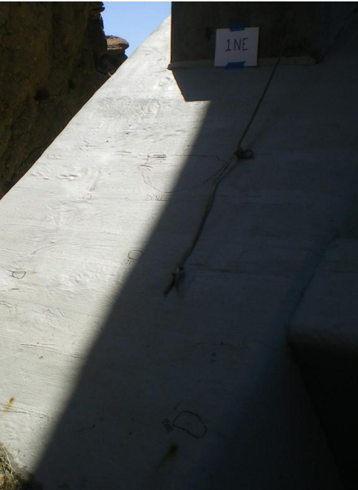
Figure A3. Bay 1NE, 5 voids
