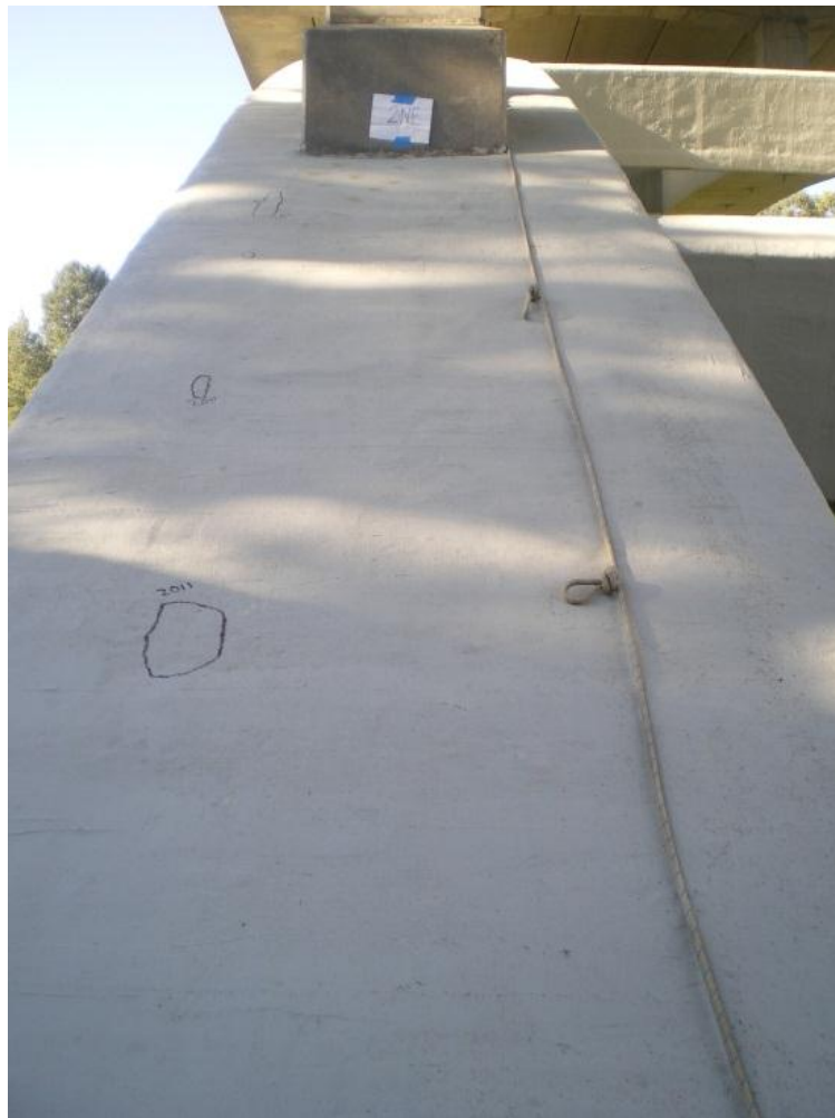
Figure A6. Bay 2NE, 3 Voids
