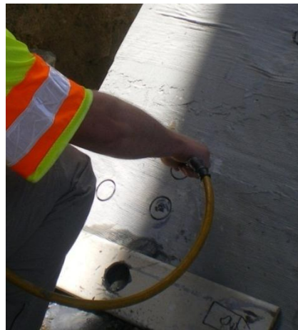
Figure 3.29. Removing water and debris from core cuts
