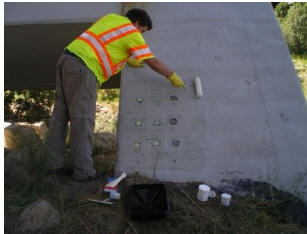
Figure 3.56. Applying a primer coat to the areas for repair
