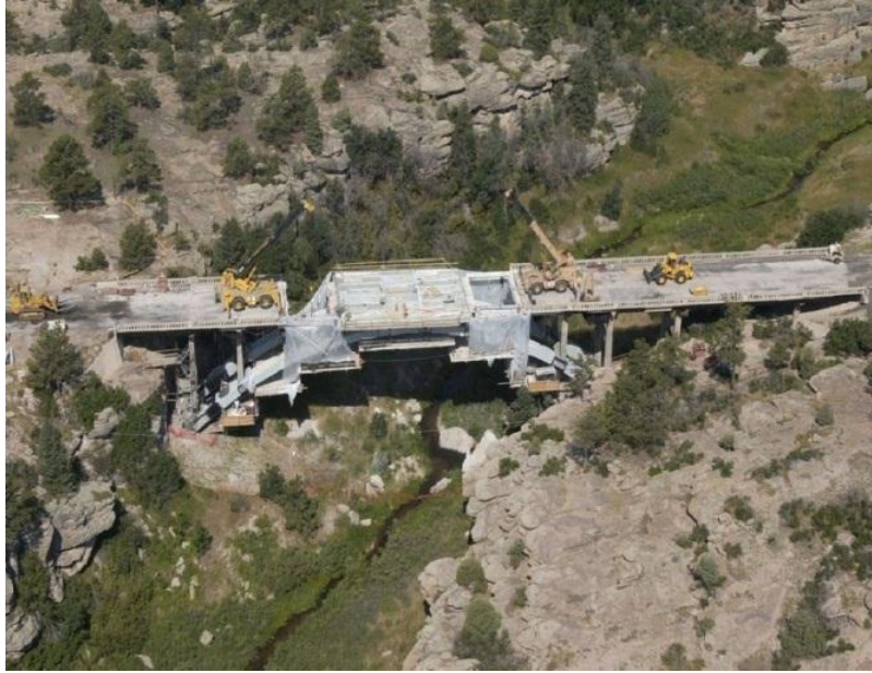
Figure 3.6. Systematically replacing the bridge deck (Mohseni, CDOT)
