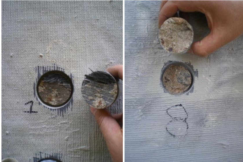
Figures 3.42 and 3.43. Failure Modes B and F: cohesive failure in FRP laminate, and mixed cohesive failure in substrate and adhesive failure at the adhesive/substrate interface, respectively (on left), Failure Mode G: cohesive failure in concrete substrate (on right)
