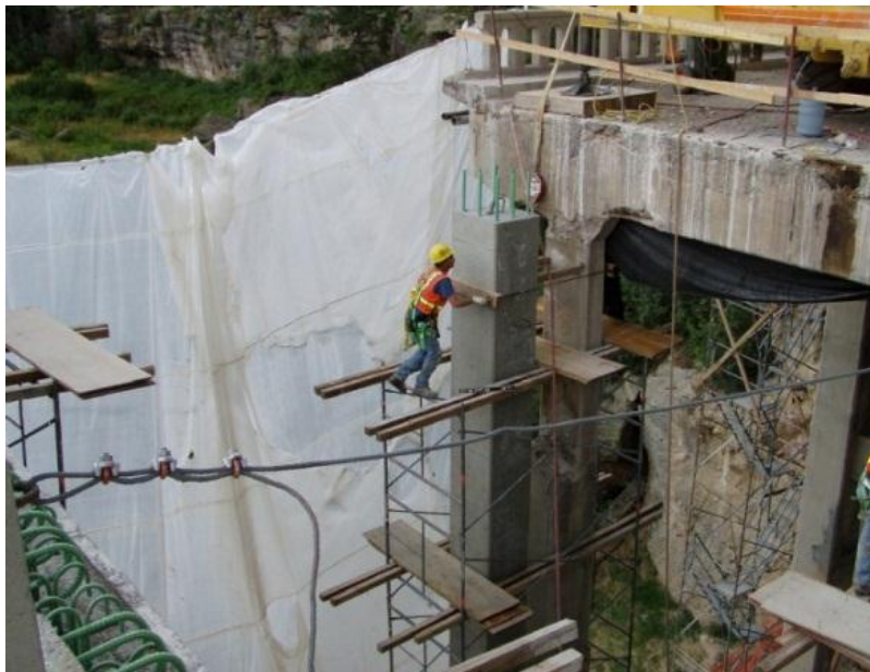
Figure 3.7. Placing the new spandrel columns adjacent to the existing columns (Mohseni, CDOT)
