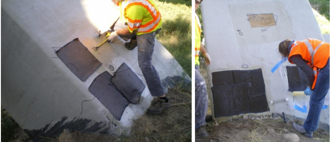
Figures 3.57 and 3.58. Allocating fabric for repair and applying the second layer of CFRP to the area of pull-off tests on the east arch
