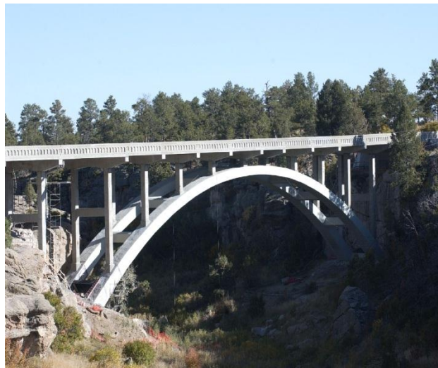
Figure 3.4. Castlewood Canyon Bridge after the 2003 repair (Mohseni, CDOT)
