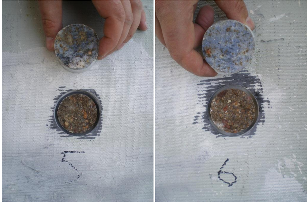
Figures B12 and B13. Test No.14, weak bond strength, and Test No.15, weak bond strength
