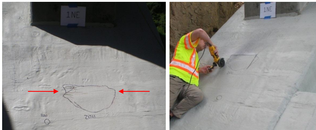
Figures 3.48 and 3.49. Void in CFRP with transverse crack identified with red arrows and Cutting the perimeter of the void in the CFRP
