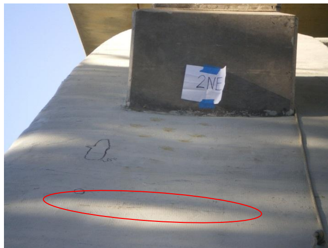
Figure 3.20. Crack identified in 2007
