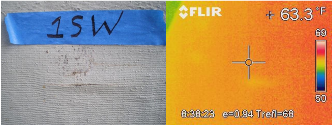
Figure A24. Photograph and thermal image of a defect found in Bay 1SW
