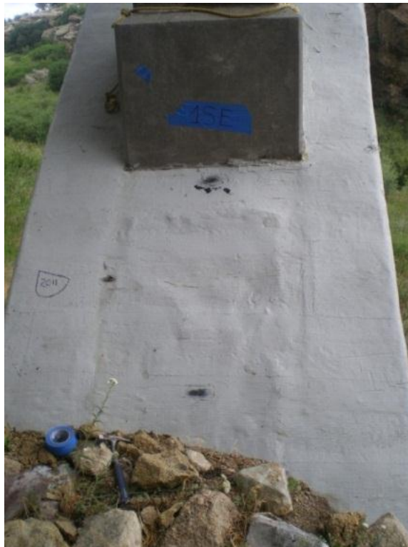
Figure A23. Bay 1SE, 1 void
