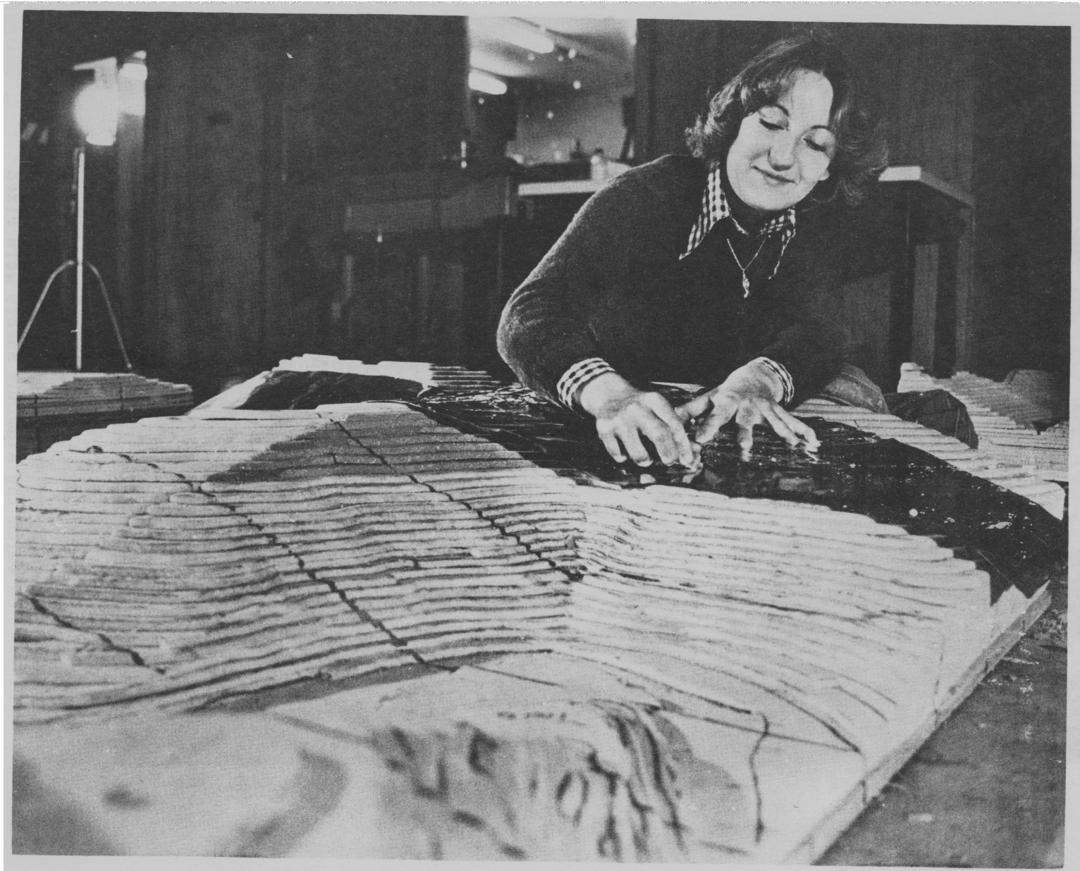
Figure 3-2. Picture Showing Technique for Constructing Aluminum Shell Model.
