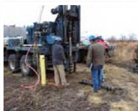
*Drilling a monitoring well (above) and the completed well (below).*
