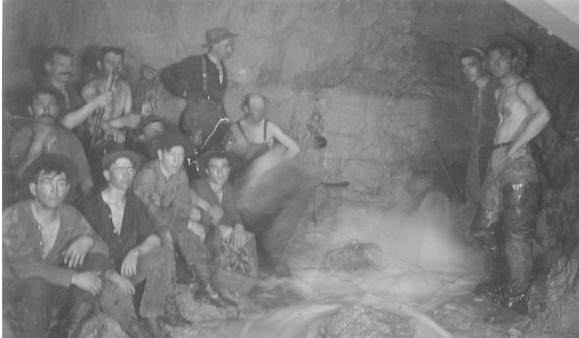
1905. These Gunnison Tunnel workers had just struck water. The water was very hot and there was as yet no ventilation shaft. The temperature in the tunnel was around 90 degrees Fahrenheit. Source: UYWUA
