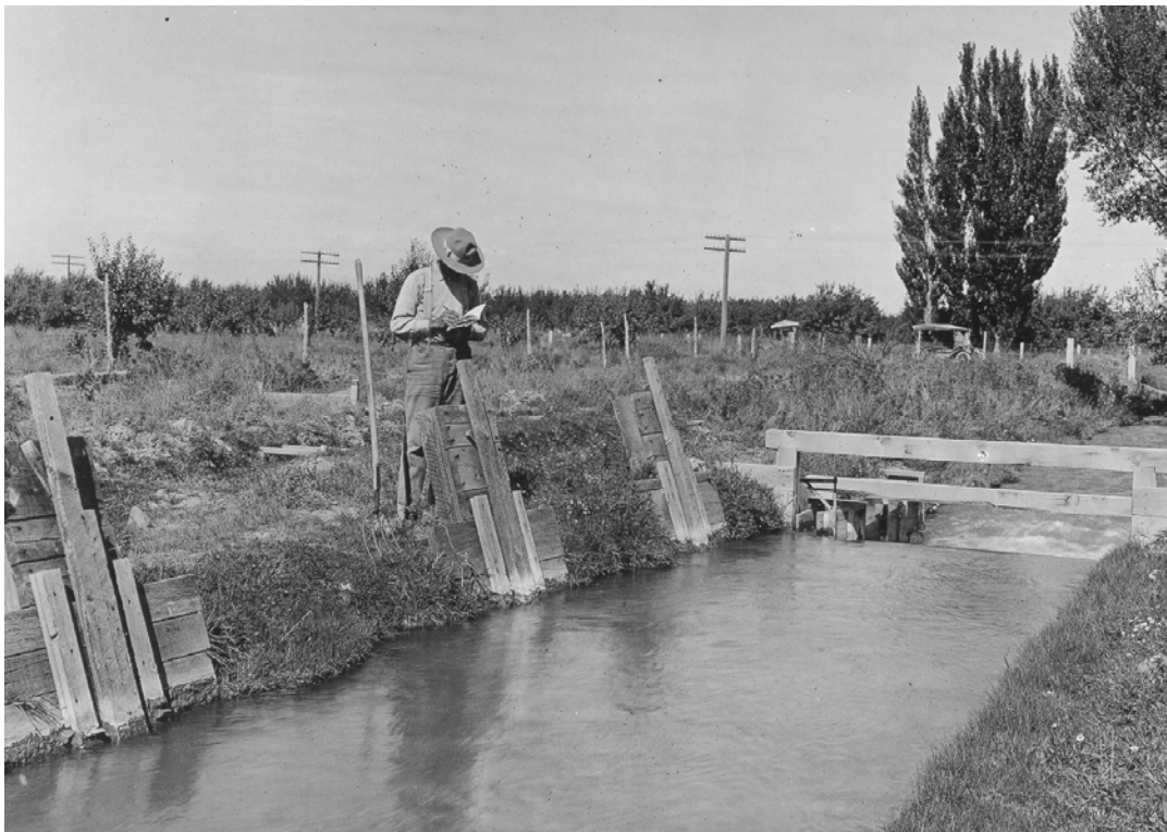
A ditchrider checking "tapbox and spillbox diversions" on Spring Creek Lateral, early 1900's, Source: UVWUA
