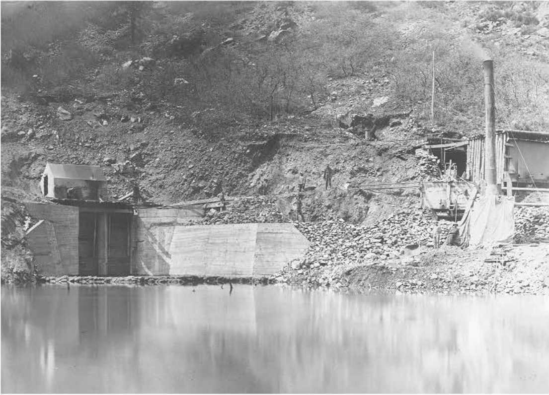
Gunnison Tunnel construction (above) and tunnel workers (below) early 1900's Source: UYWUA
