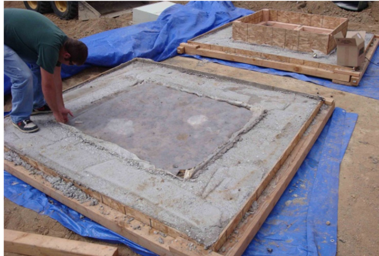
Figure 4.9 Expansive soil-rubber field plots post compaction, prior to the application of vertical seating stress and subsequent inundation
