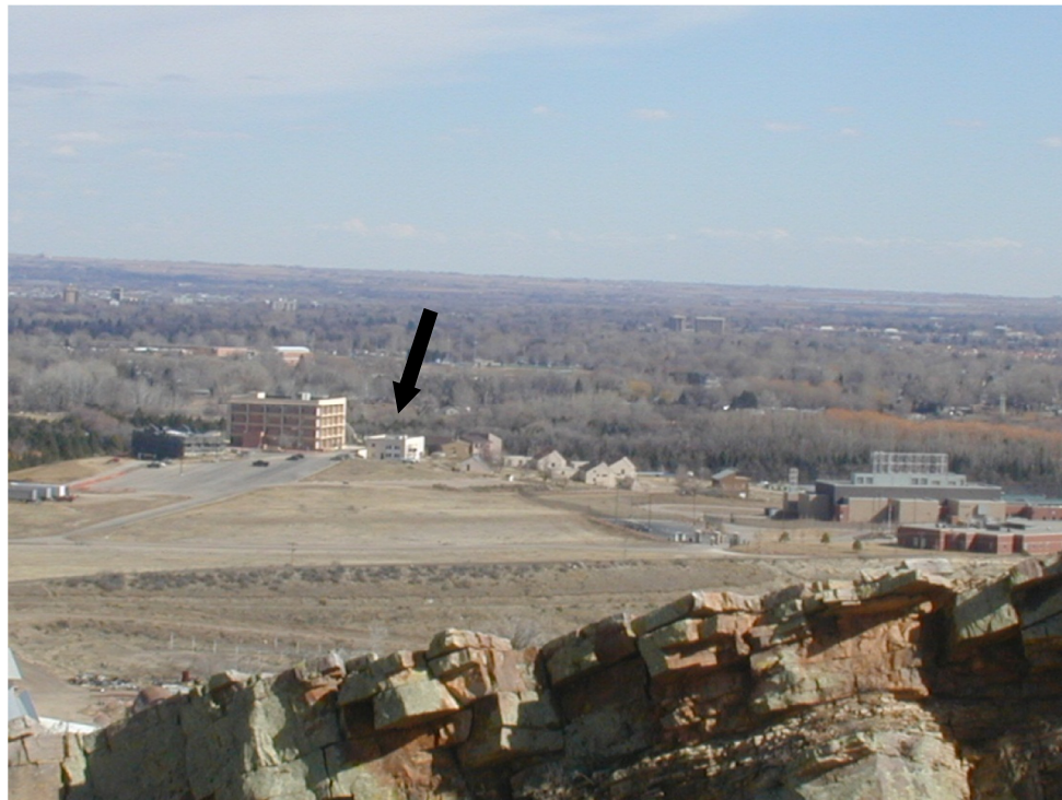
Figure D.2 Photograph of the ESTS looking East southeast (after Benvenga 2005)
