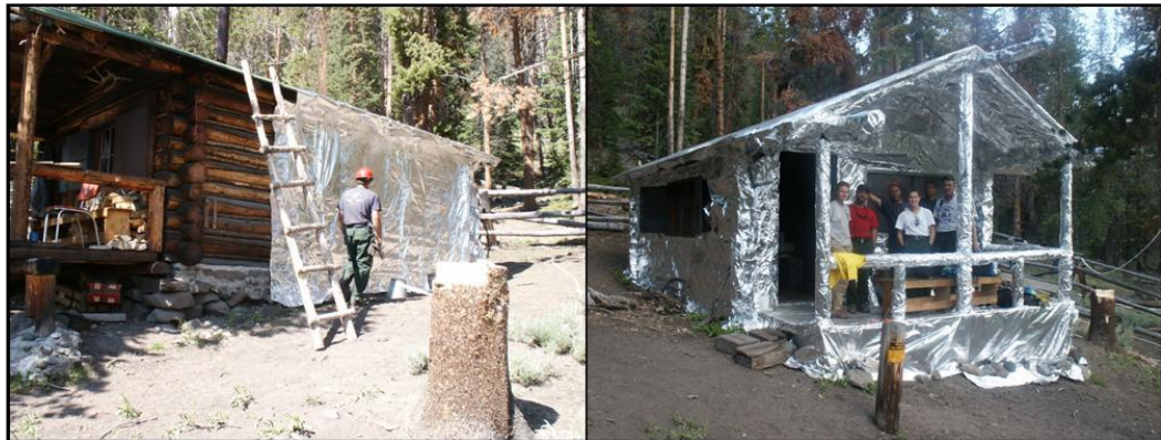
Figure 1.5. Example of one of the management strategies. The crew seen above is protecting the Venus Cabin from the LVF. This building survived. This image was adopted from the 2006 Case Review, Little Venus Fire Shoshone National Forest WY-SHF-09.
