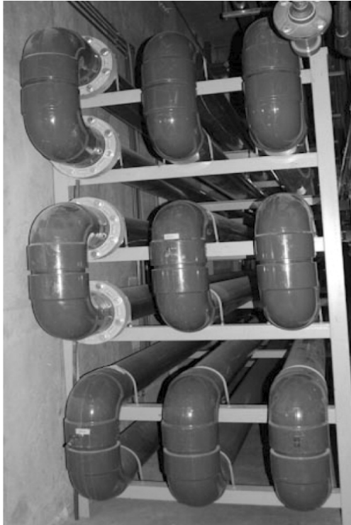
Figure 2. Pipe loop (from Wilson and Venayagamoorthy, 2010)
