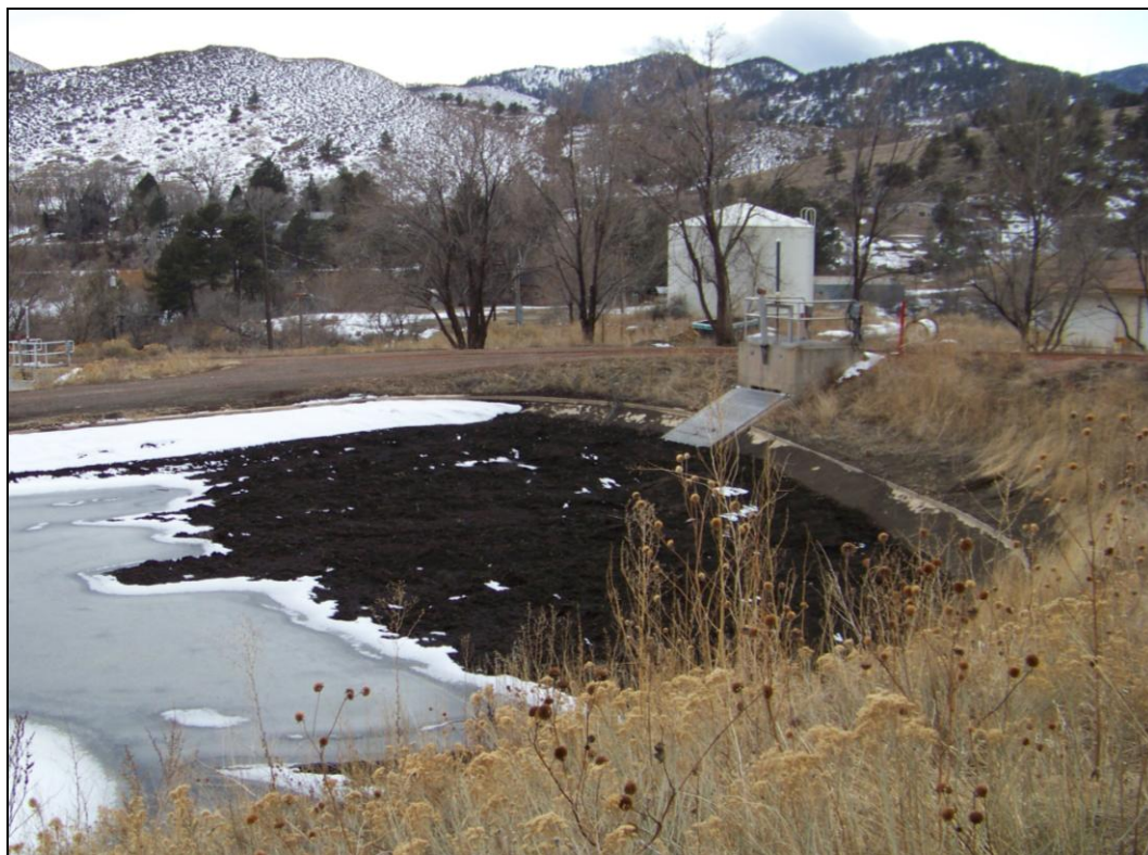
Figure 3-2 Al-WTR solid in a sludge drying basin
