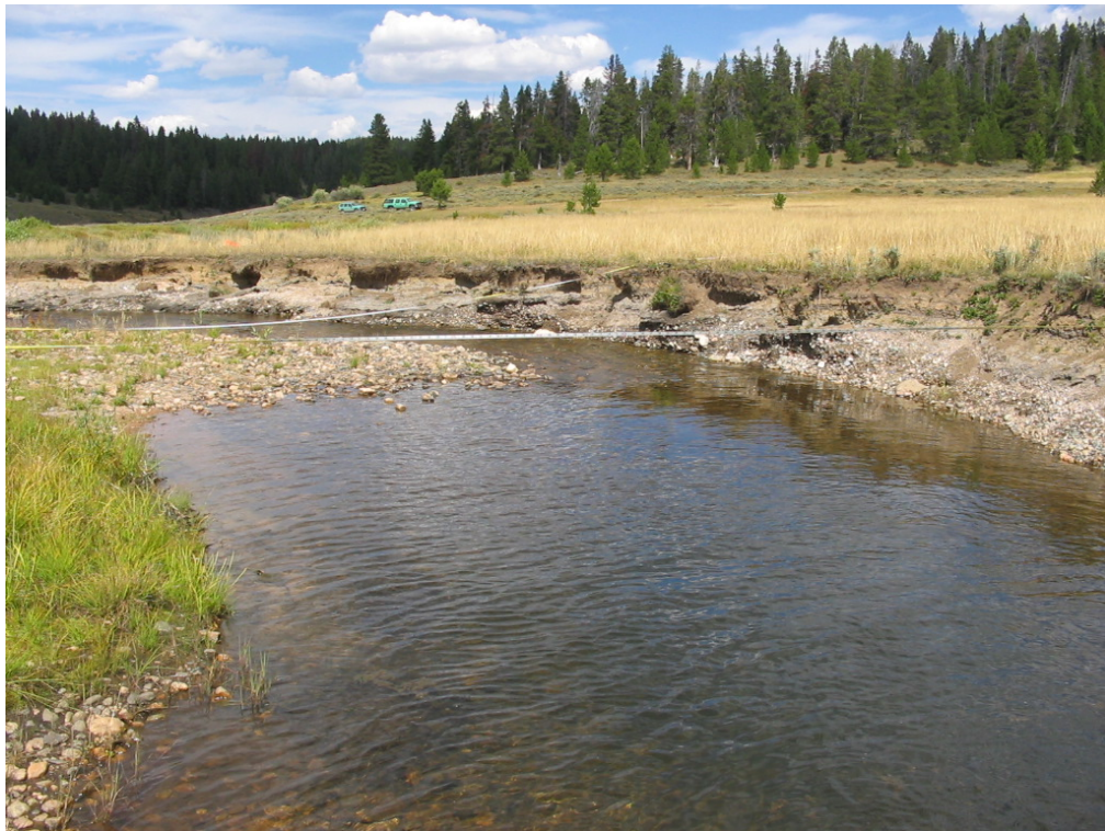
Figure A.37: Erosion along outside of meander bend in Site 4, 2007 (photo by D. Cenderelli).
