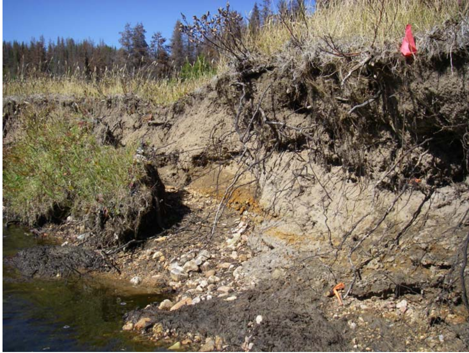
Figure A.13: Bank erosion in Site 2, 2008.
