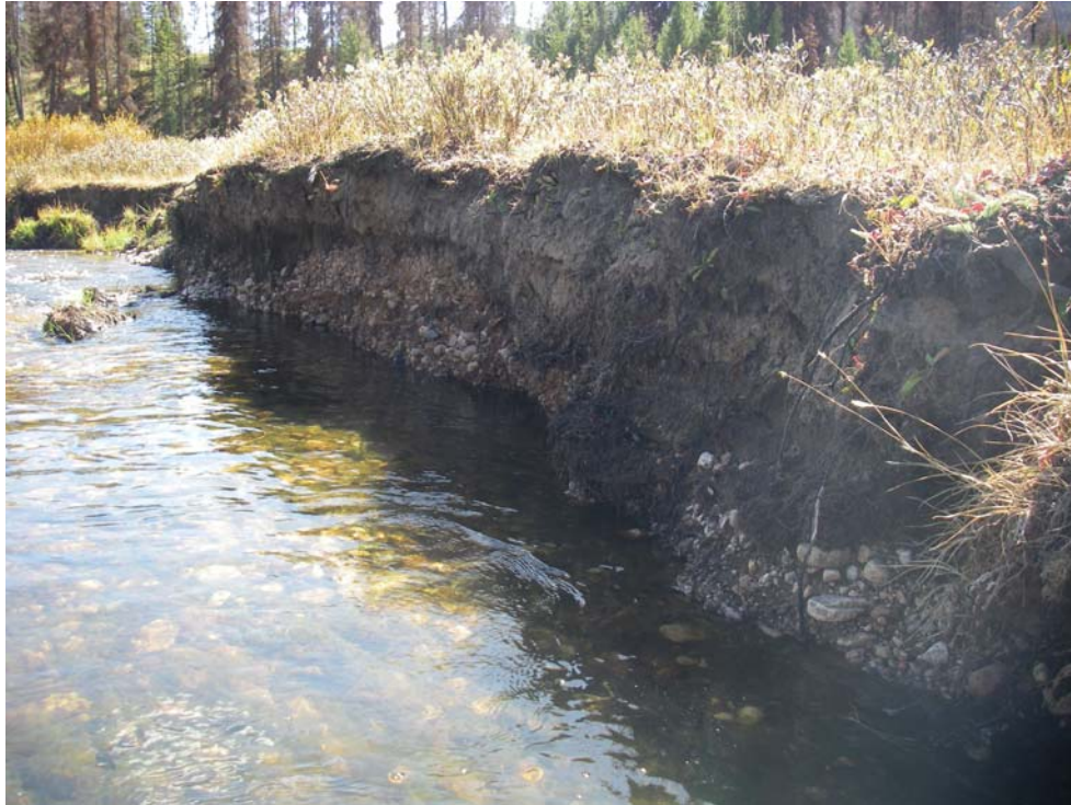
Figure A.27: Bank erosion in Site 3 at low summer base flow, 2008.
