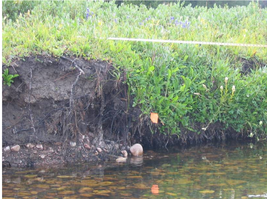
Figure 4.30: Photo of partially failed bank in site 2.
