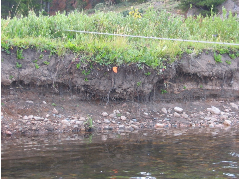
Figure A.15: An example of slumping in Site 2, 2008. A tension crack exists in the bank top. The orange flag indicates an erosion pin location, indicating a cross section, also is located here.
