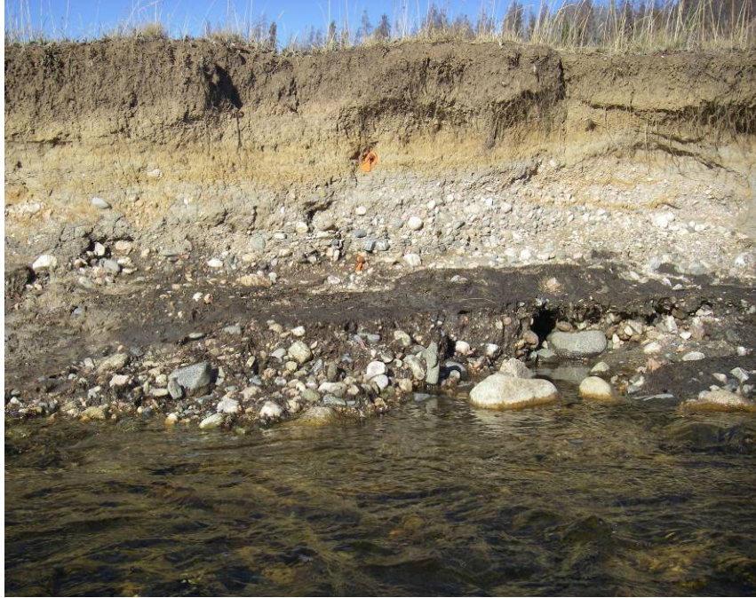
Figure 3.2: Example of the placement of two erosion pins in a vertical bank. The bank is located in a meander bend in Site 4, pins are indicated by orange flagging.
