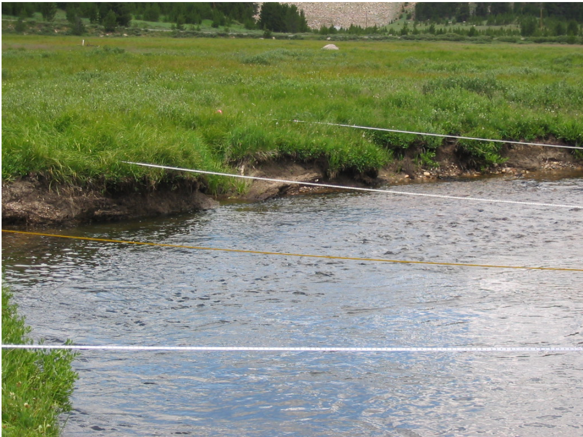
Figure A.7: typical bank erosion along right bank in Site 1, 2007. Photo by D. Cenderelli.
