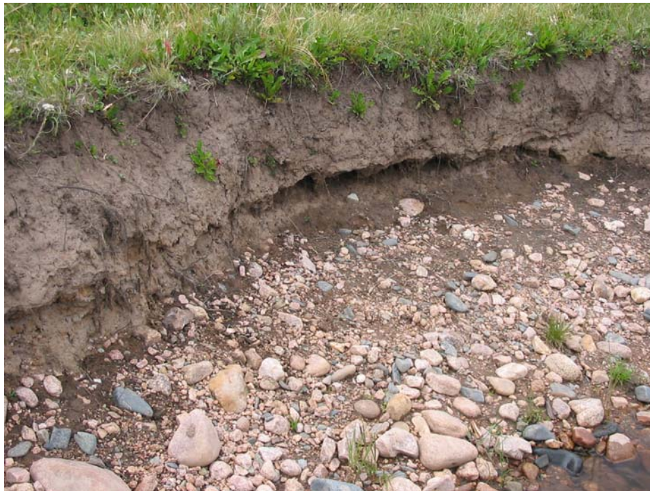
Figure A.14: Bank erosion along right bank in Site 2, 2009. Note the coarser gravel deposit at the toe, and preferential erosion occurring mid-bank.
