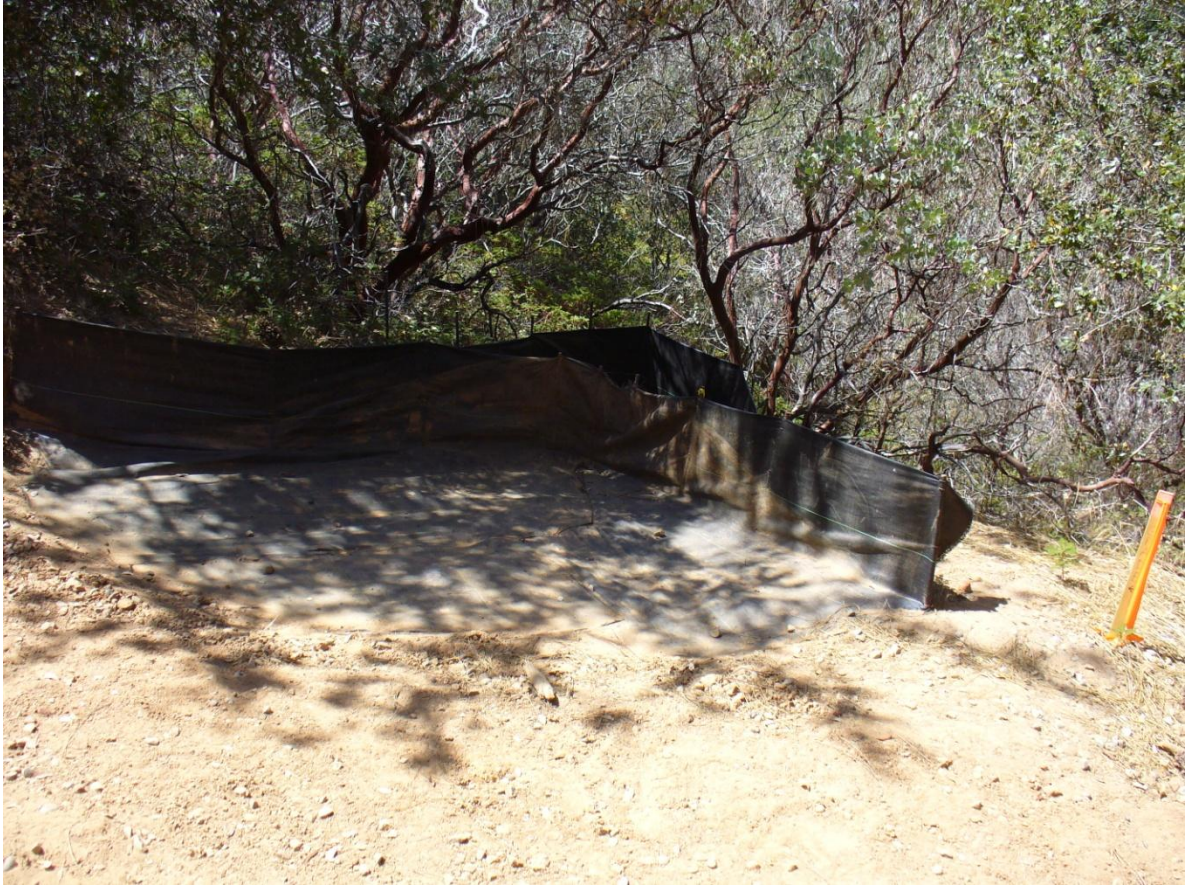
Figure 3.4. One or more sediment fences were installed at the drainage point of road segments in José Basin and the Providence Creek watersheds. The fence in the foreground was installed in summer 2007 in José Basin just below a waterbar draining a native surface road segment, and the second fence was added in summer 2008 to prevent overtopping.
