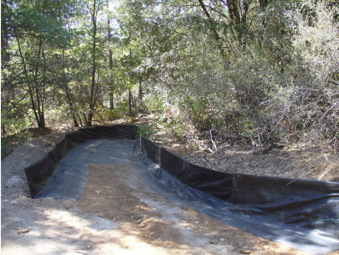
Figure 2.6. Sediment fences were installed at the drainage point of native surface road segments in José Basin as well as the Providence Creek and Bull Creek watersheds. This fence was installed just below a waterbar draining a native surface road segment in José Basin in summer 2007.
