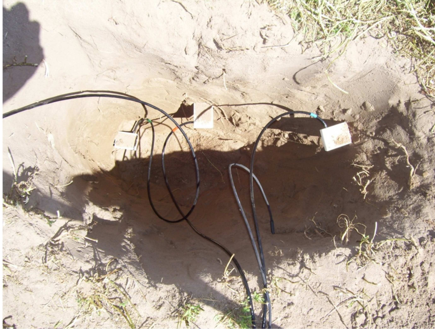
Figure 9. CS625 Sensors Installed at Depths of 30-, 61-, and 91-cm.
