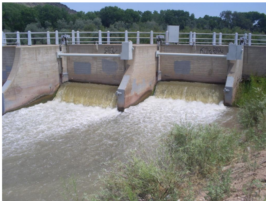
Figure 4.2 Albuquerque Main Canal Heading at Angostura Dam
