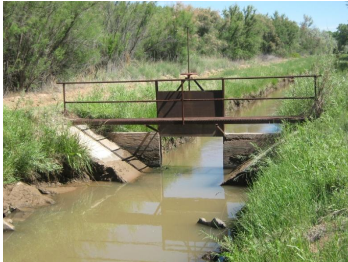
Figure 4.3 A Typical Check Structure in an Open Position
