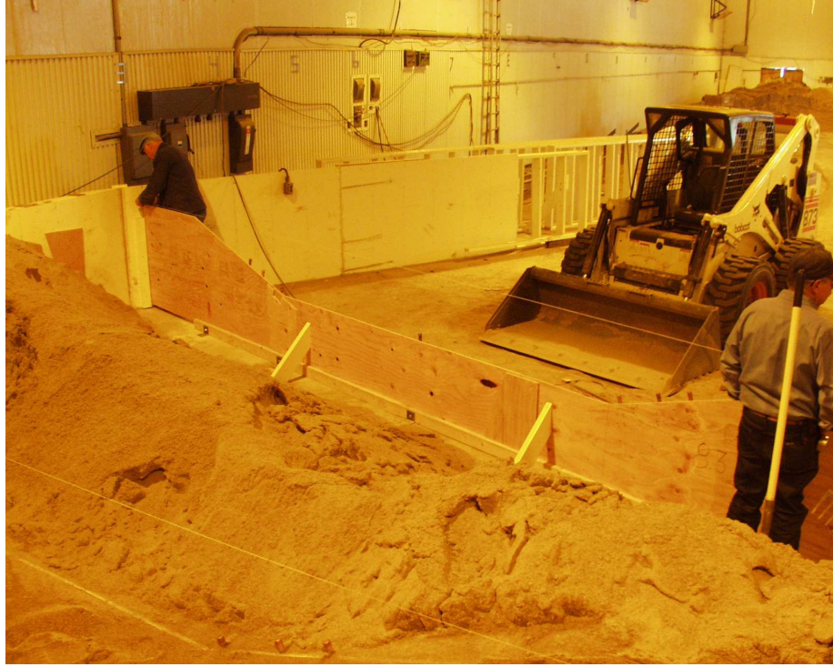
Figure A.6 Skeleton of the Main Channel and Filling Material of Main Channel
