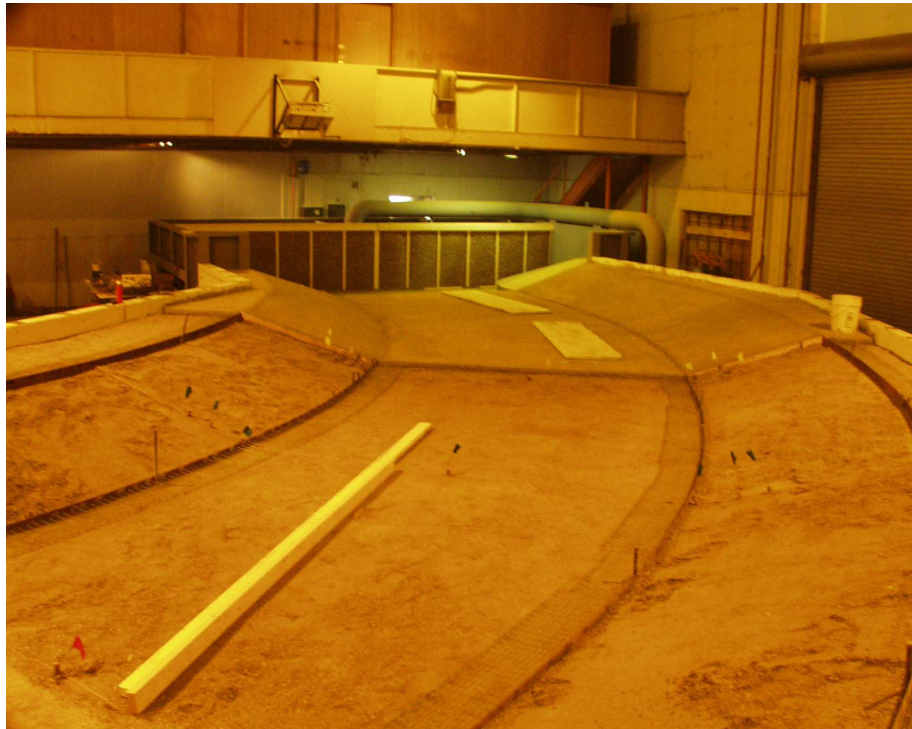
Figure A.8 Installation of Steel Flashing
