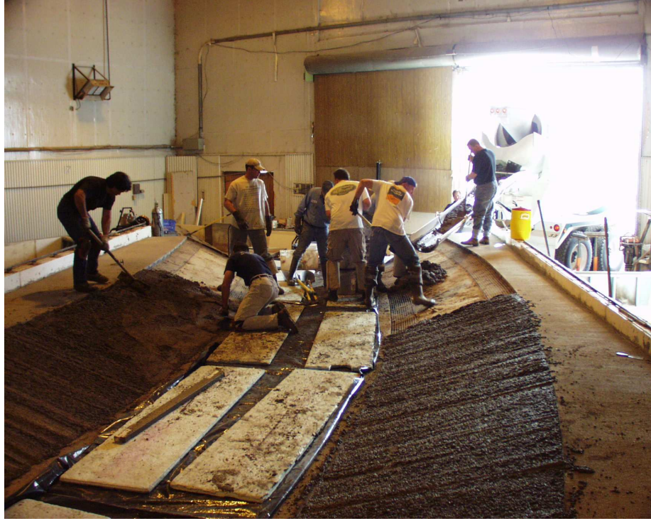
Figure A.9 Concrete Placement for Model Construction
