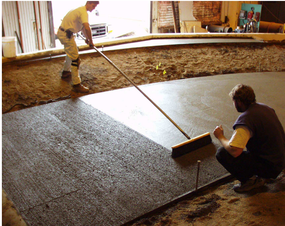
Figure A.10 Concrete Broom Finish for Desired Channel Roughness
