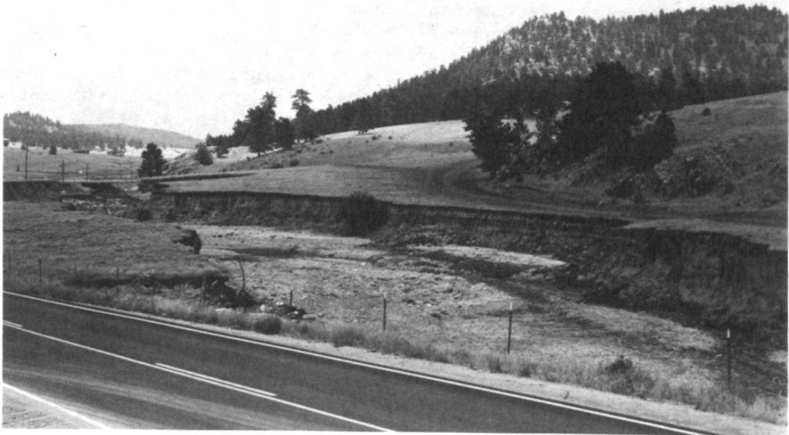
FIGURE 62 Erosion along Dry Gulch
