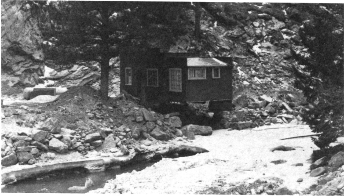
FIGURE 51 Erosion of Foundation Bearing Material
