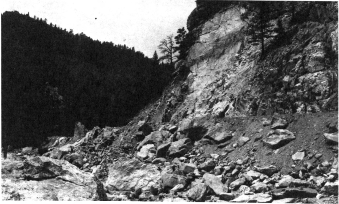
FIGURE 56 Rock Fall along Highway
