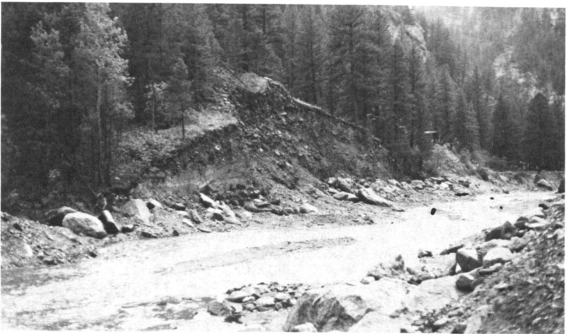
FIGURE 63 Erosion of Debris Fan
