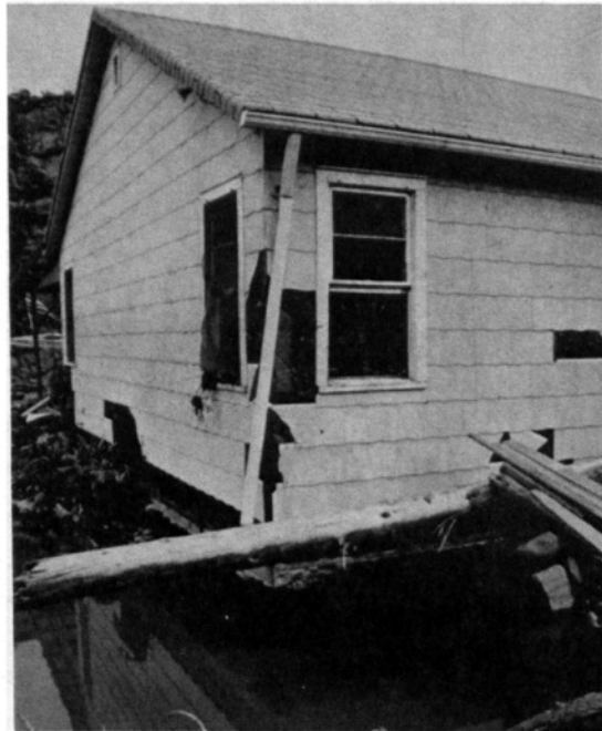
FIGURE 54 Erosion below Slab on Grade Foundation
