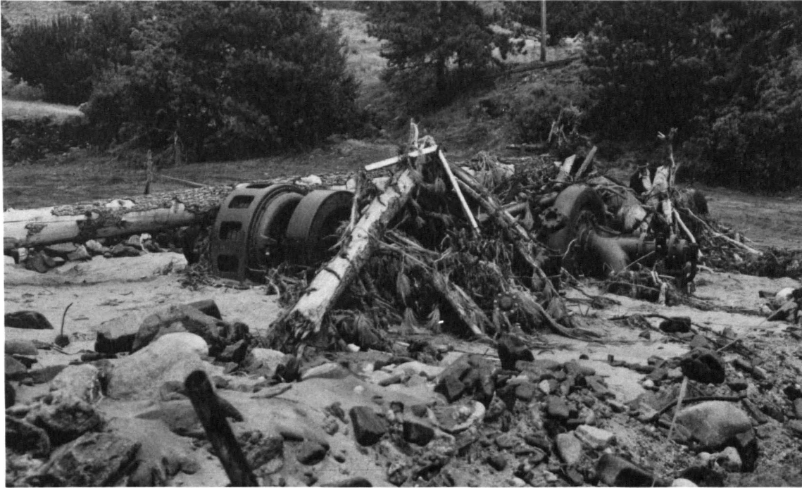
FIGURE 69 Remains of Loveland Power Plant at Loveland Mountain Park
