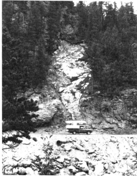
FIGURE 57 Landslide in Residual Soil
