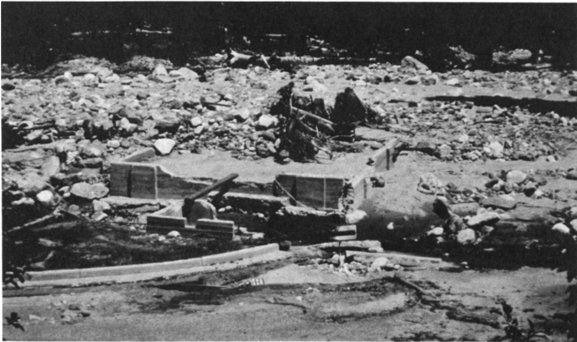
FIGURE 48 Loveland Power Plant
