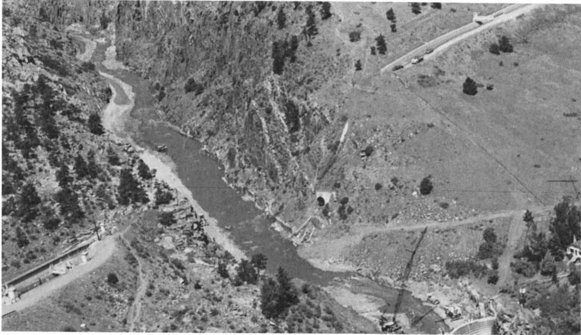
FIGURE 70 Siphon Support Structure and Feeder Canal Located at the Mouth of the Canyon
