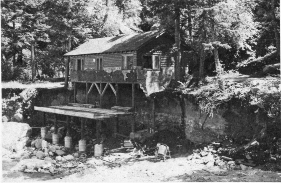
FIGURE 53 Remedial Measures Being Taken for Foundation Repair
