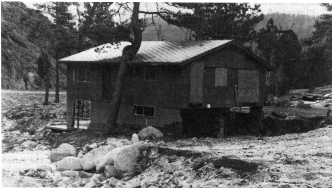
FIGURE 50 Failure of Concrete Block Foundation
