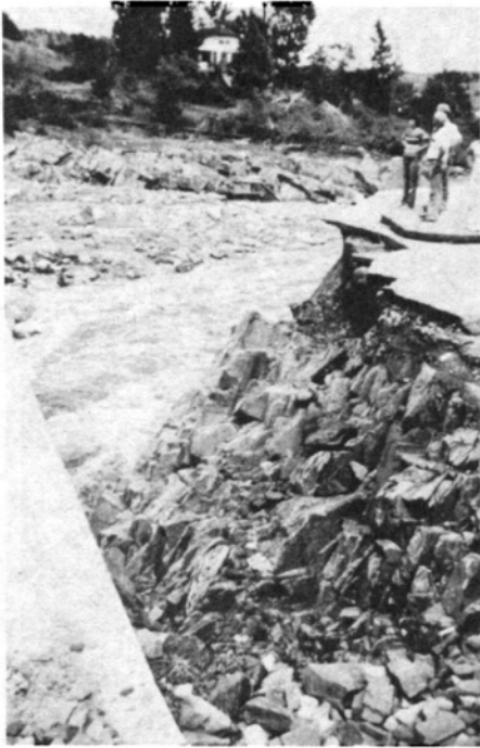
FIGURE 40 Erosion of Backfill Material at Bridge Abutment
