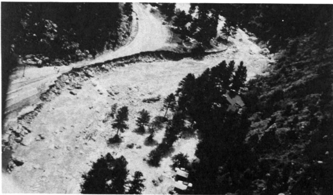
FIGURE 36 Erosion of Outside Bend on U.S. Highway 34
