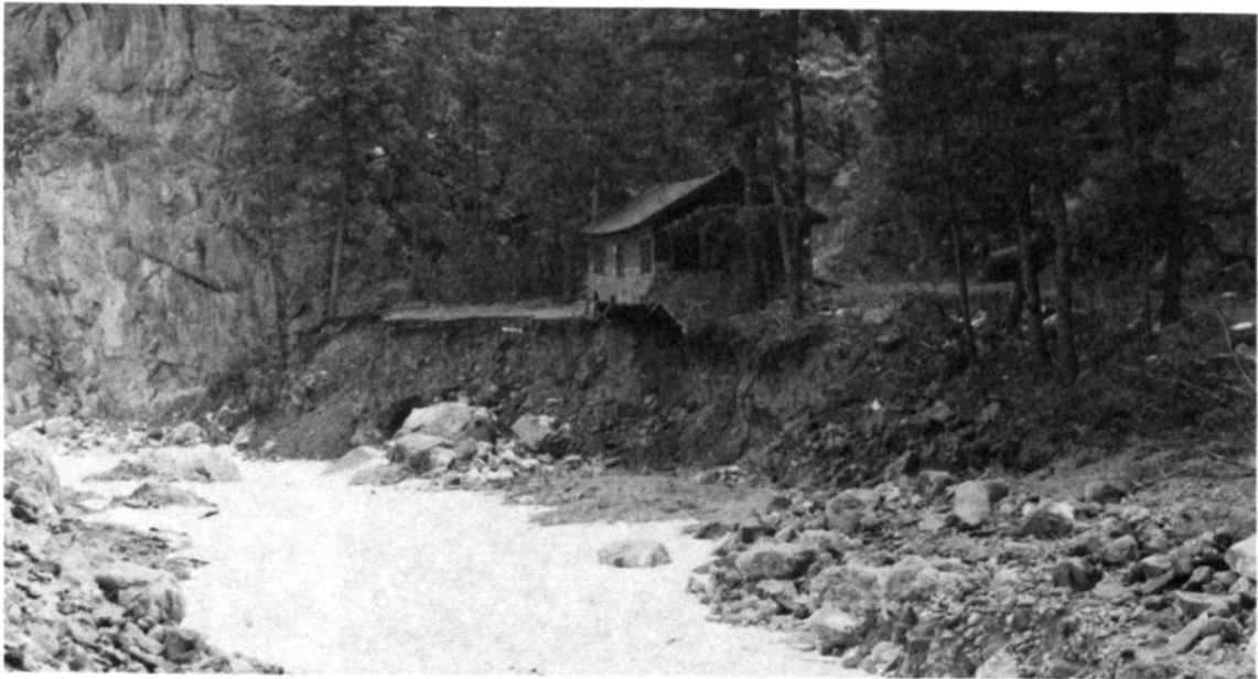
FIGURE 52 Erosion of Debris Fan below Foundation
