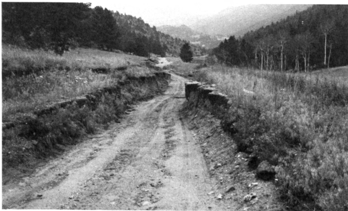
FIGURE 39 Extensive Gullying in Dunraven Glade Area
