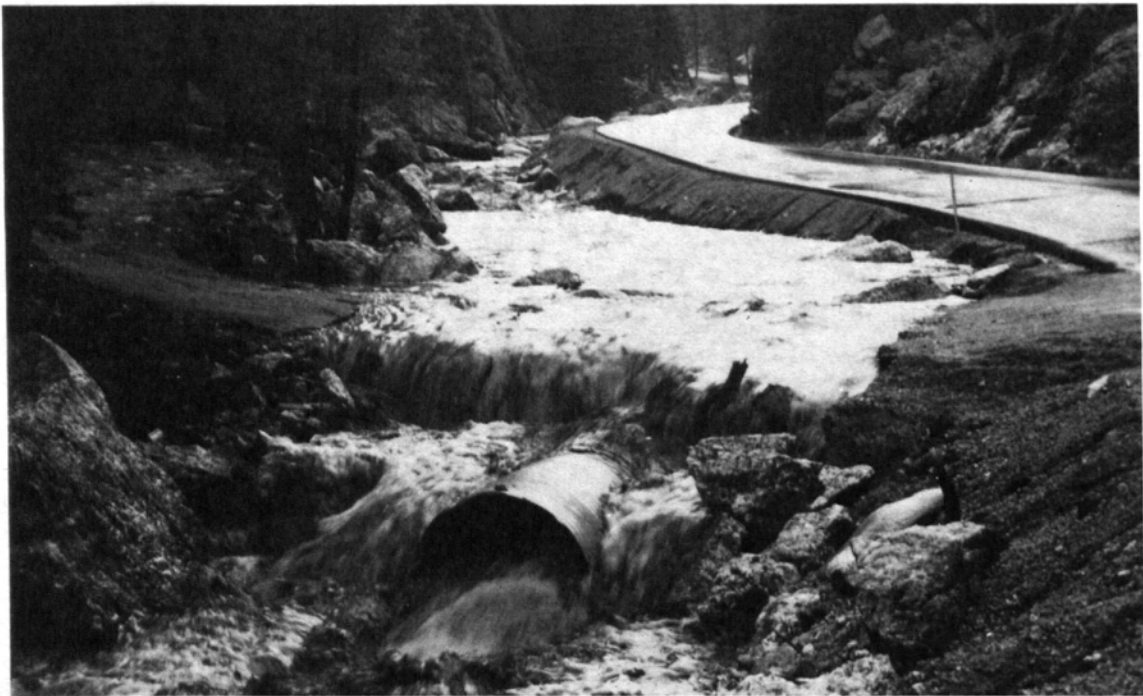
FIGURE 46 Storm Waters Washing over Culvert
