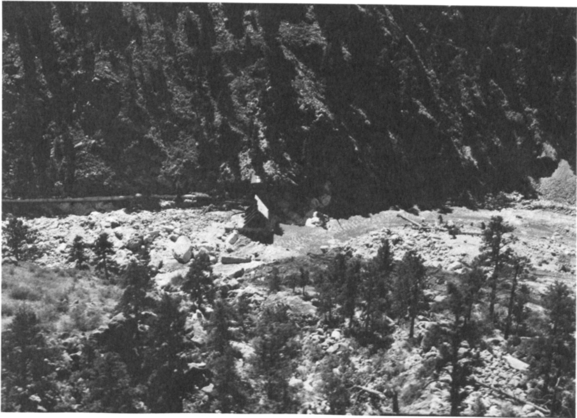
FIGURE 64 Remains of Loveland Hydroelectric Dam
