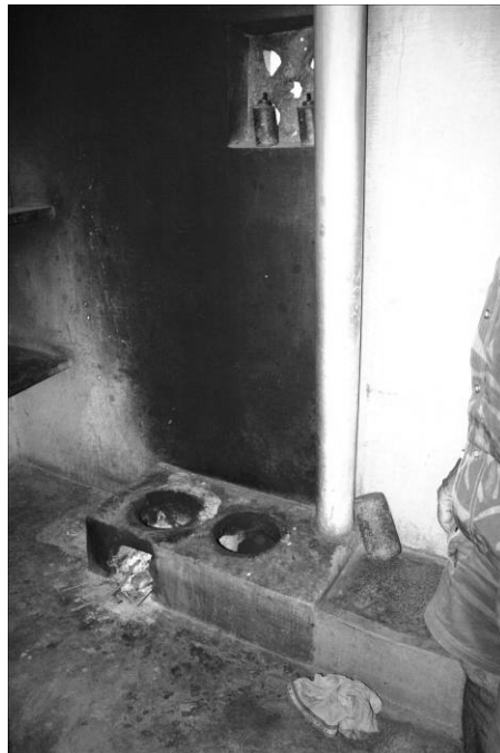
Figure 1. A home in India with walls blackened by PM from biomass combustion 9
