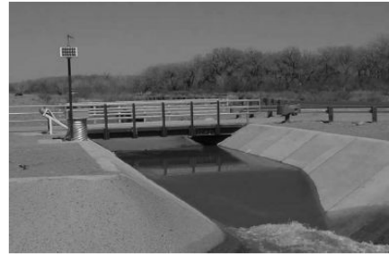
Fig. 2. Broad crested weir gauging station with radio telemetry
