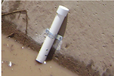
Figure 4: Installed Hobo Pressure Transducer
