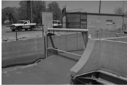
Fig. 3. Langemann gate used as a canal heading
