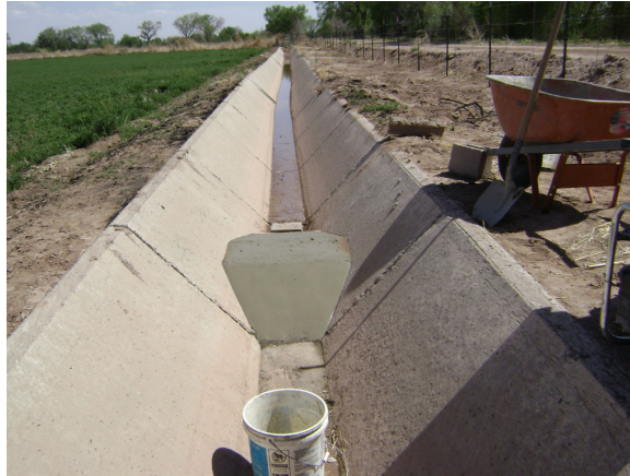
Figure 2: Completed Broad Crested Weir for Field 3
