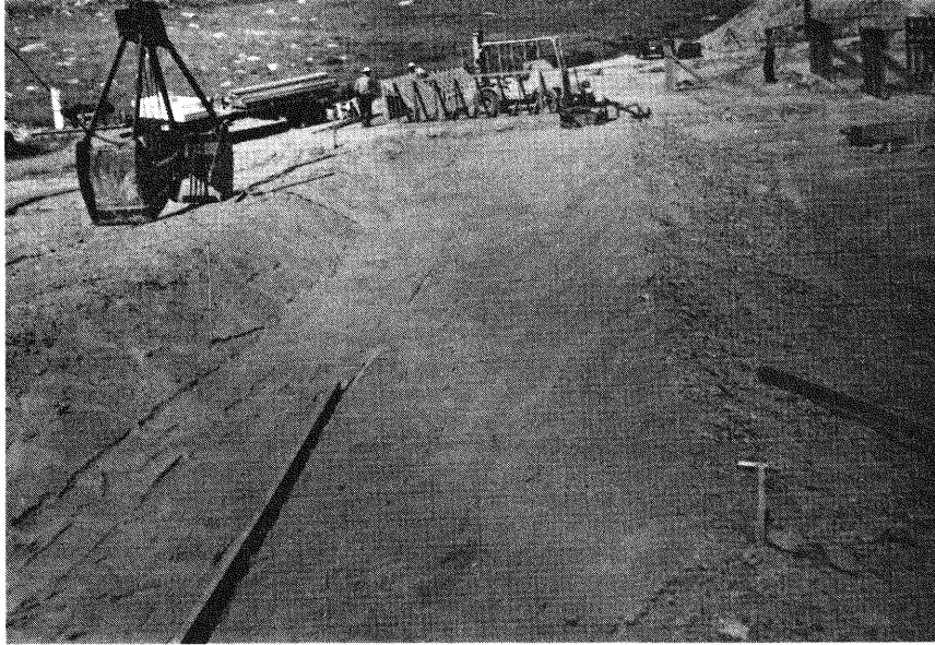
FIGURE 8: CLOSE-UP OF EXCAVATION: Approximately 3 feet deep x 8 feet wide x 80 feet long.
