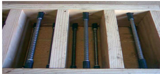
Fig.3.10: Timber forms and rebar for corrosion specimens
