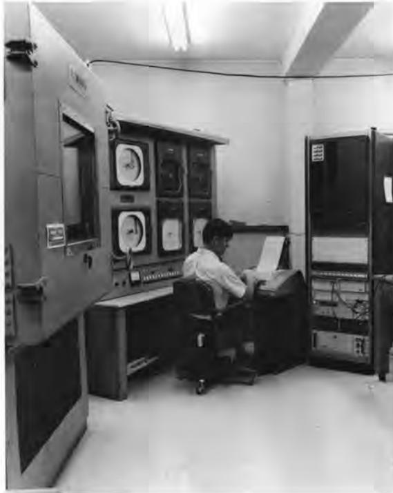
Figure 72. NCAR Computer-Controlled Environmental Chamber. The one-cubic-meter chamber is on the left and the computer controller is on the right. Photo courtesy of NCAR.
