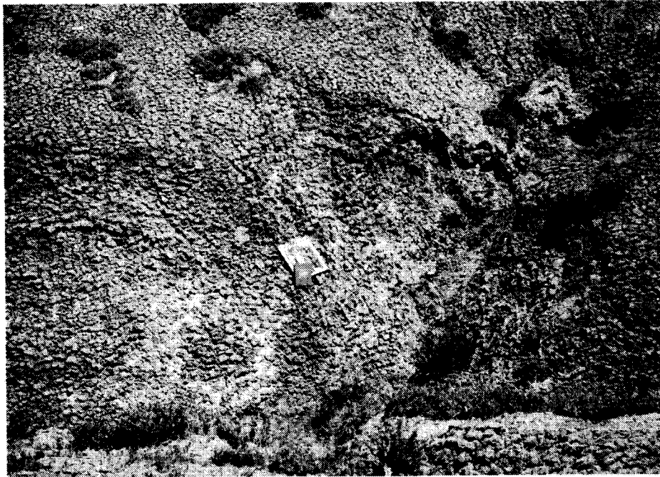
Fig. 5.6. Gravity-induced slope failure.
