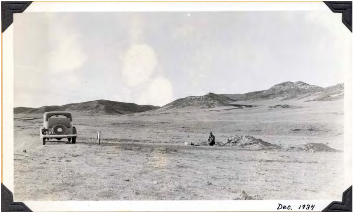
Figure 32. Major Coffin in an excavation pit on top of the hillslope in December 1934.
