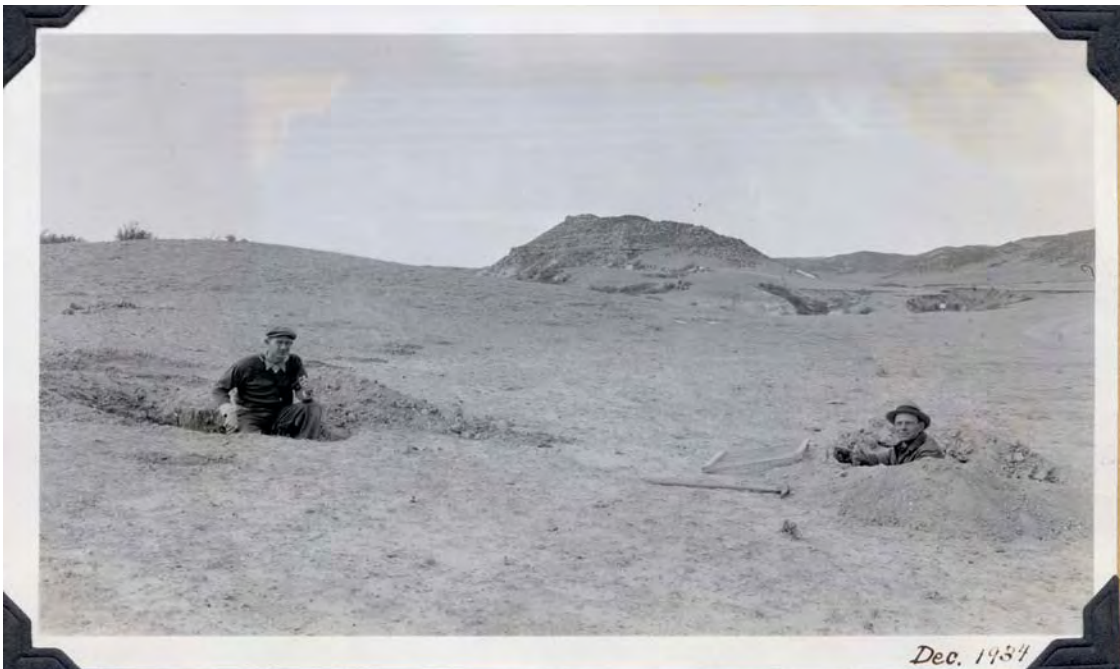
Figure 31. A. Lynn Coffin and Judge Coffin in two excavation pits on top of the hillslope in December 1934.
