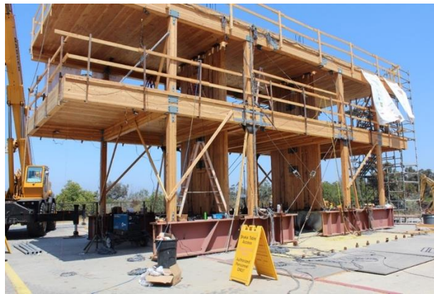
Figure 3: Two-story CLT building with post-tensioned rocking walls
