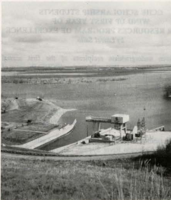
Kingsley Hydroelectric Generating Plant
