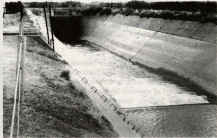
Inverted siphon at Paxton carries water to Seminole Reservoir
