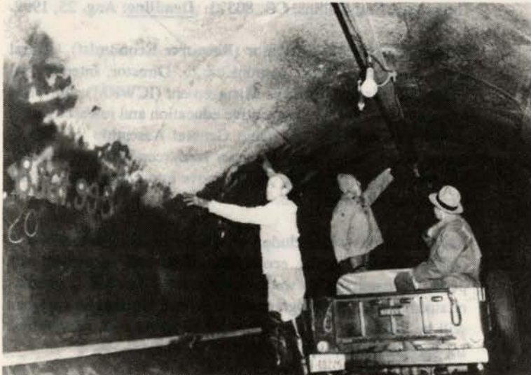
CBT Staff Inspect the Alva B. Adams Tunnel - 13.1 miles in length, 9 ft. 9 and 3/4 inches in diameter
