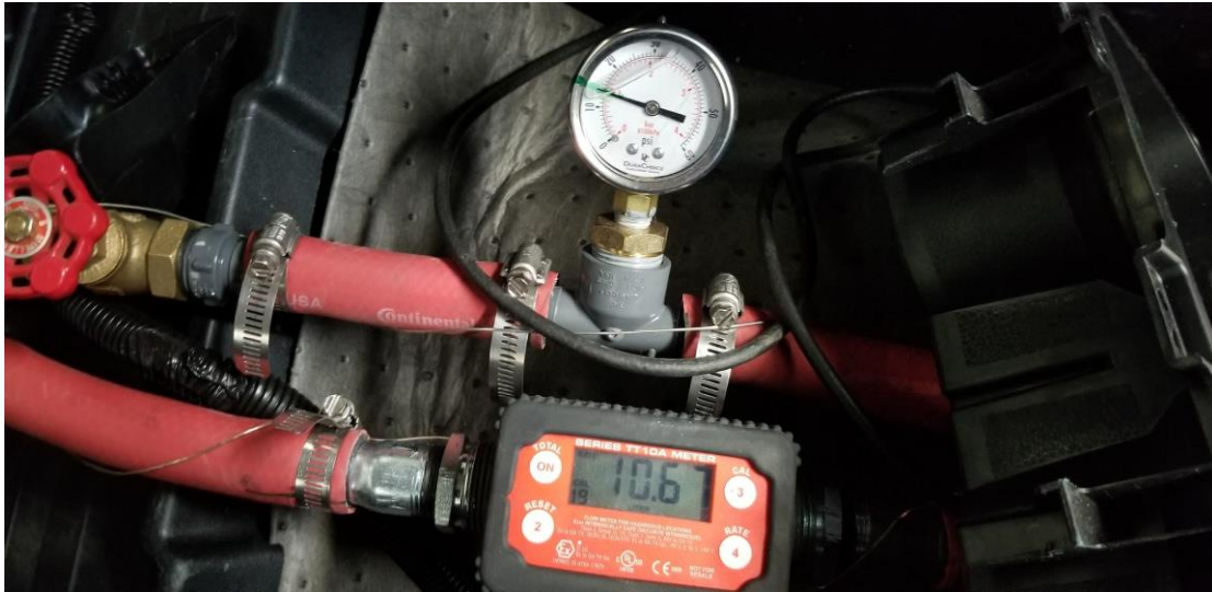
Figure 46: Tested oil flow rate, LPM
