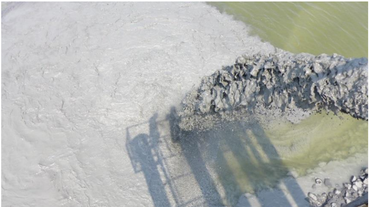
Figure 2 The discharge of the mud mixture into the Porong River at the Pejarakan Outlet
