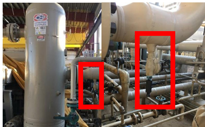
Figure 43: Inlet Gas Sampling Point (upstream of compressor scrubber)
