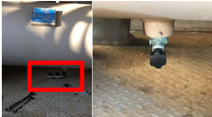
Figure 44: Discharge bottle sampling point
