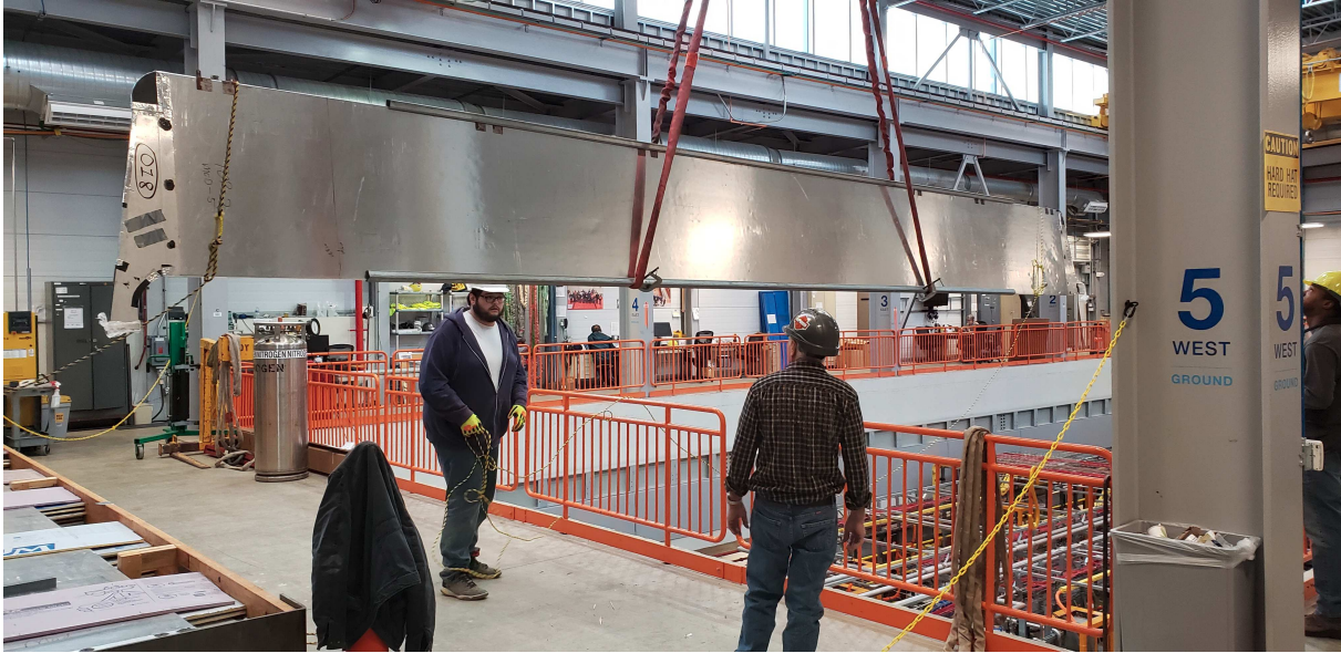
Figure 3.45: From left to right: T. Boone, J. Judd, and K. Hardin work to install the next MINOS module into the West Rolling Wall.
