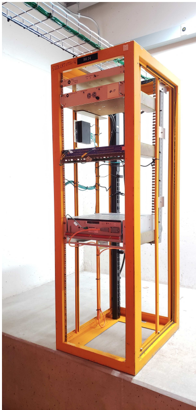
Figure 3.42: The Side CRT West Utility Rack is pictured just before the rack’s enclosure panels were added.
