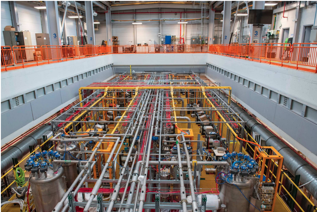
Figure 2.10: ICARUS just before the start of cold commissioning.
