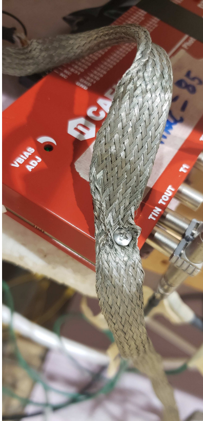
Figure 3.35: A direct ground connection to the FEB common was important to avoid electrical noise.
