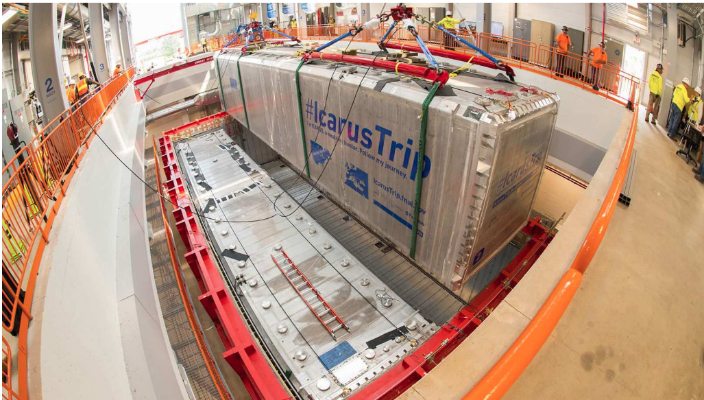
Figure 2.8: ICARUS cold vessels being installed into the warm vessel at Fermilab.
