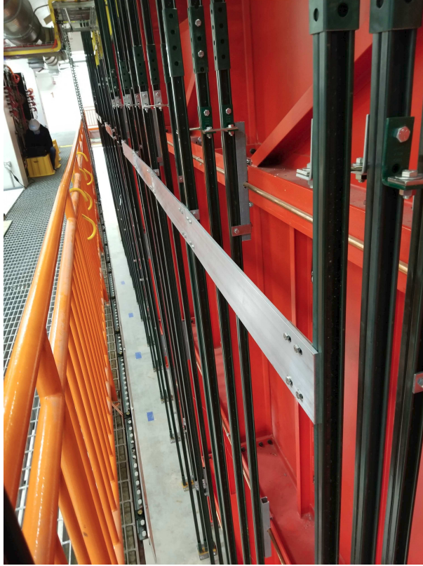
Figure 3.44: Stabilizer plates for the Side CRT West Rolling Wall can be seen on either side of the gap between the mezzanine and the Warm Vessel.
