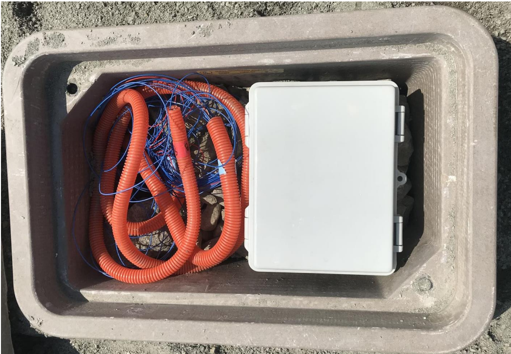
Figure A23. Photo of the inside of the field OBB electrical enclosure.
