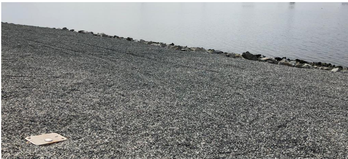
Figure 19. Photo of the field site after OBB installation.
