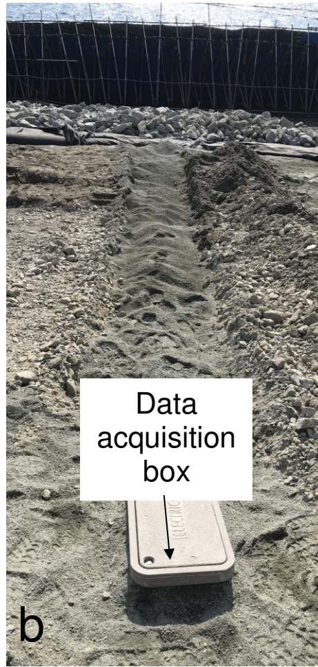
Figure 18. Photos of a) exposed and b) buried conduits leading to the data acquisition box.
