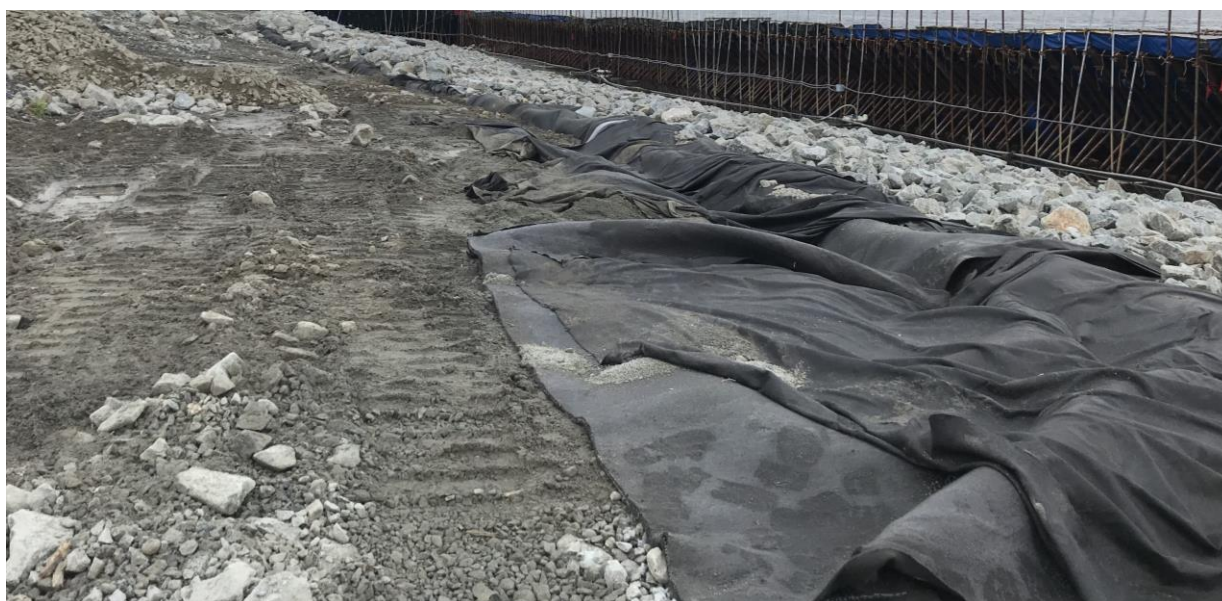
Figure A21. Photo of field OBB site.
