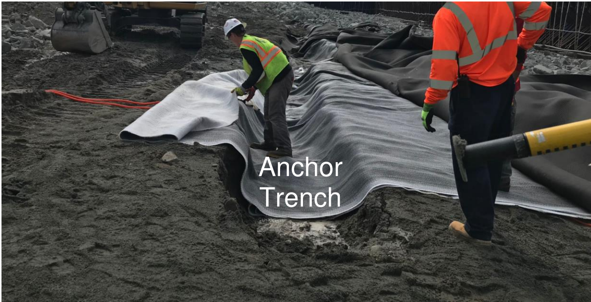
Figure 16. Photo of OBB anchor trench.
