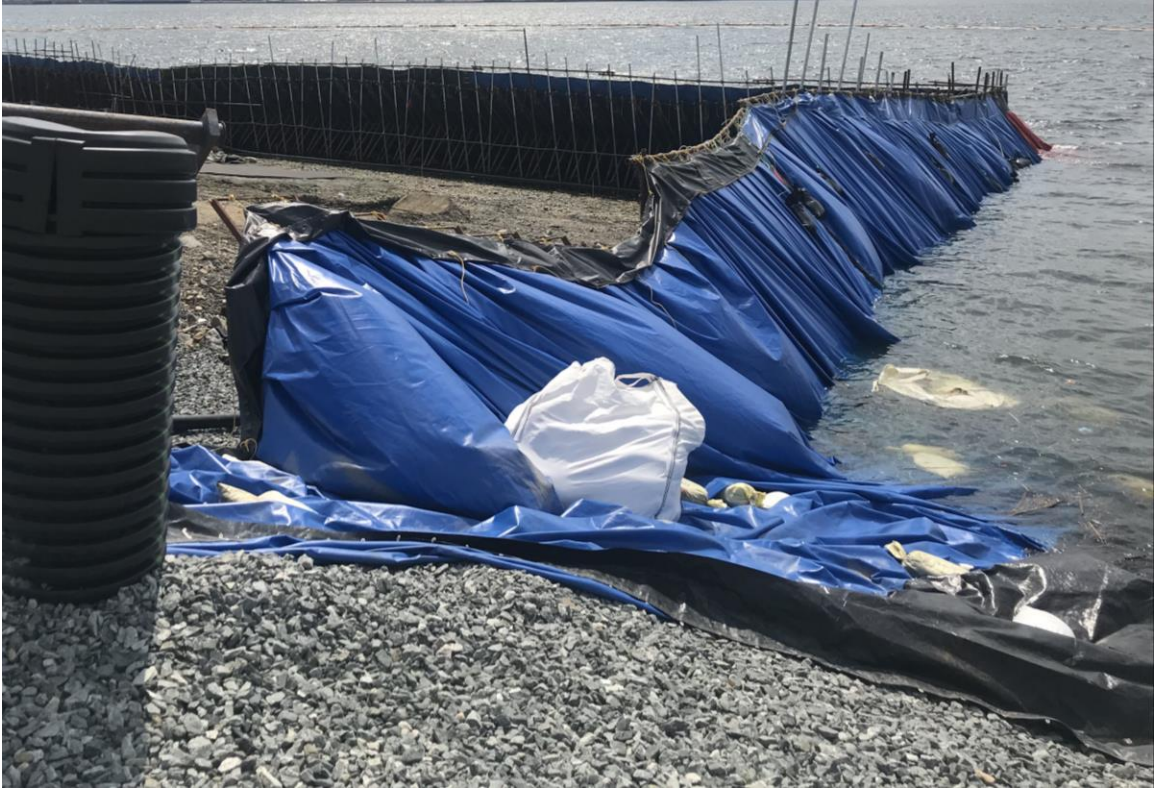
Figure A22. Photo of field OBB cofferdam.
