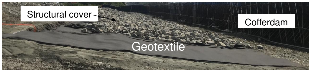
Figure 17. Photo of geotextile and structural cover layers of OBB.
