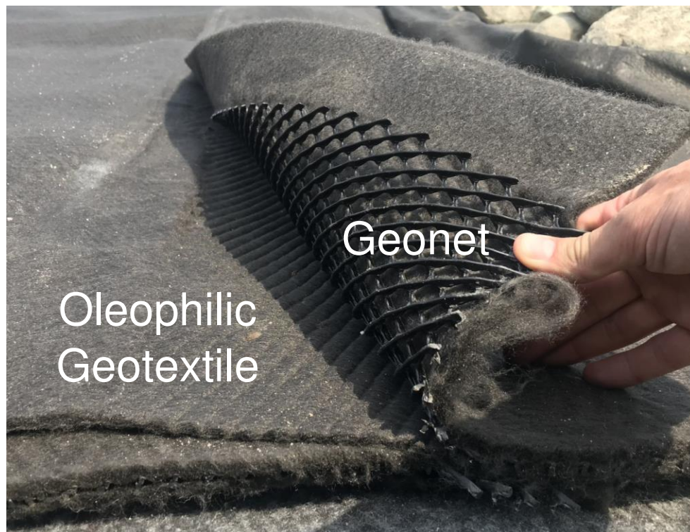
Figure 2. Photo of a geocomposite drainage layer during OBB installation.
