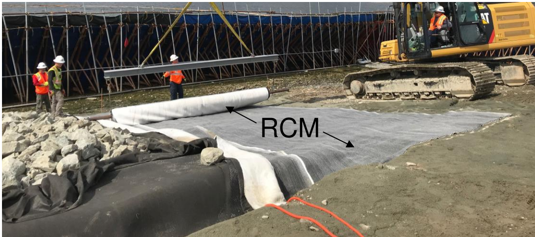
Figure 12. Photo of the RCM installation.
