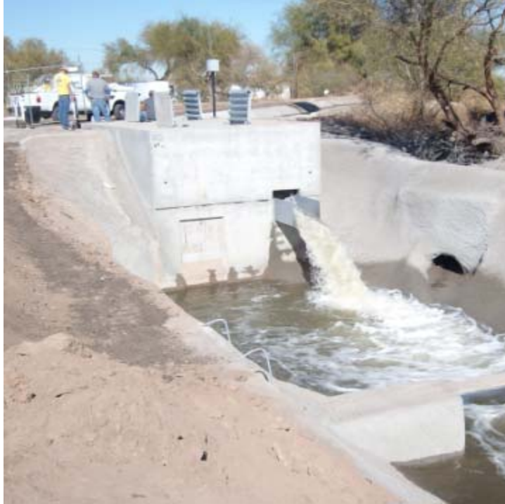
Figure 3. Installed Powerhouse – South Extension
