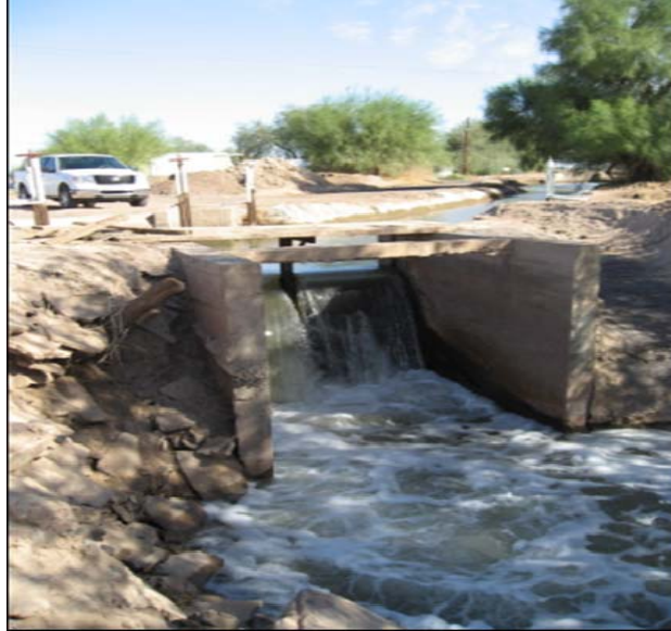
Figure 2. South Extension canal drop
