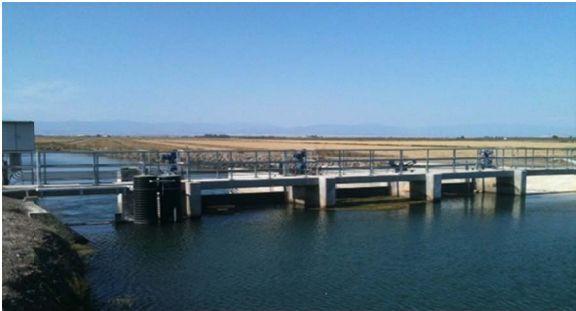
Figure 3. Typical check structure along the main canal; SCADA allows the radial gates to move automatically, maintaining a selected or targeted upstream water elevation.
