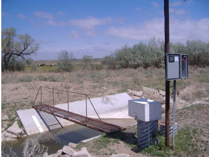
Figure 3. New Ramp-Type Long-Throated Flume at the SPDC G2 Site
