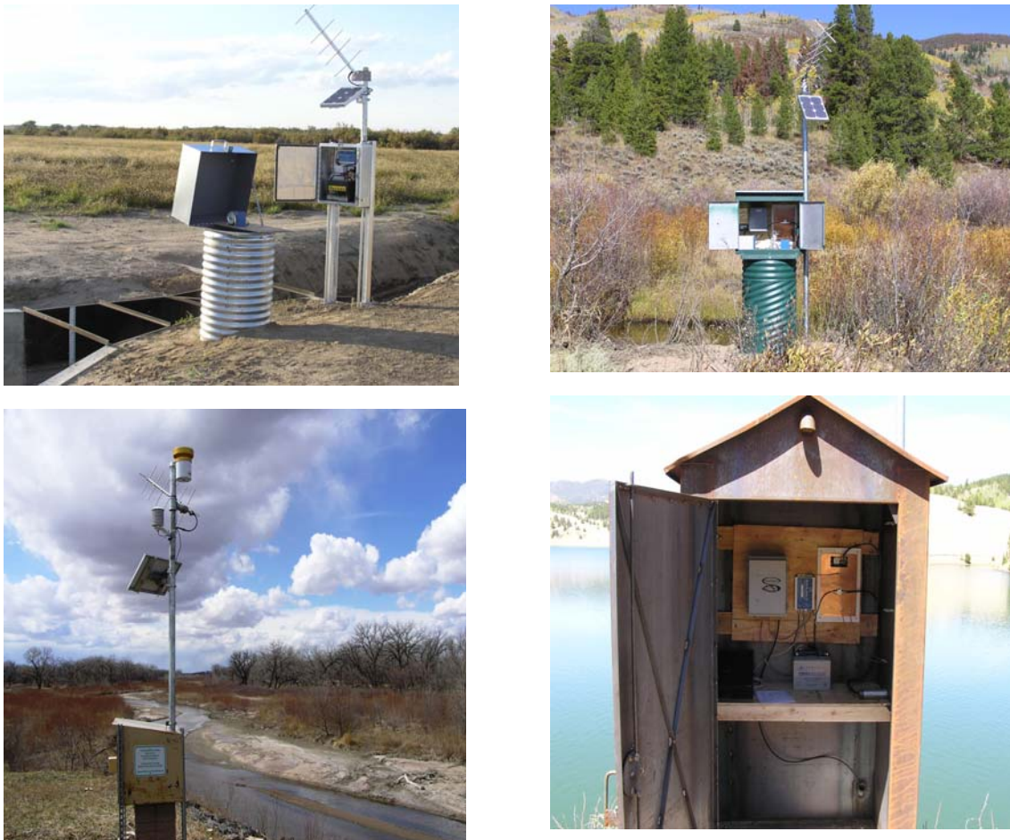
Figure 2. Photos of CO DWR gaging stations showing equipment upgrades.
