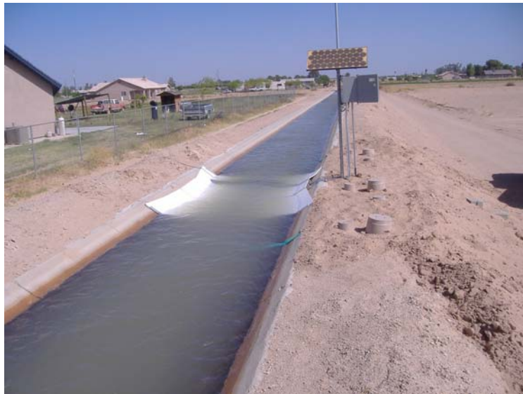
Figure 4. Unit B District Flume
