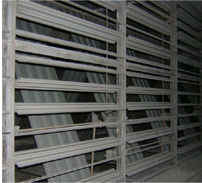
Air Dampers inside AHU
