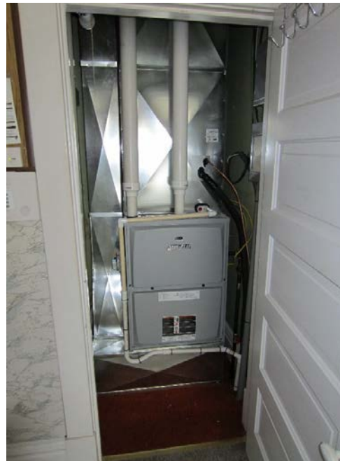
Down-Flow (Main floor closet)
