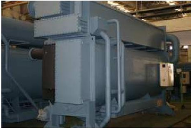
Direct-Fired SIZE: up to 1,500 tons
