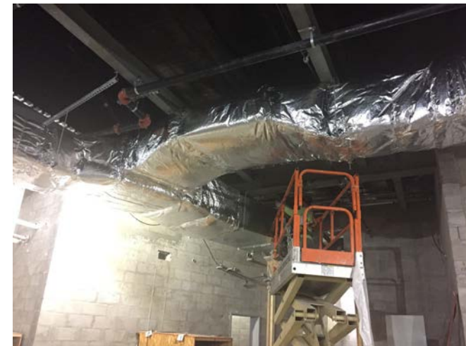
Exterior Insulated Ductwork
