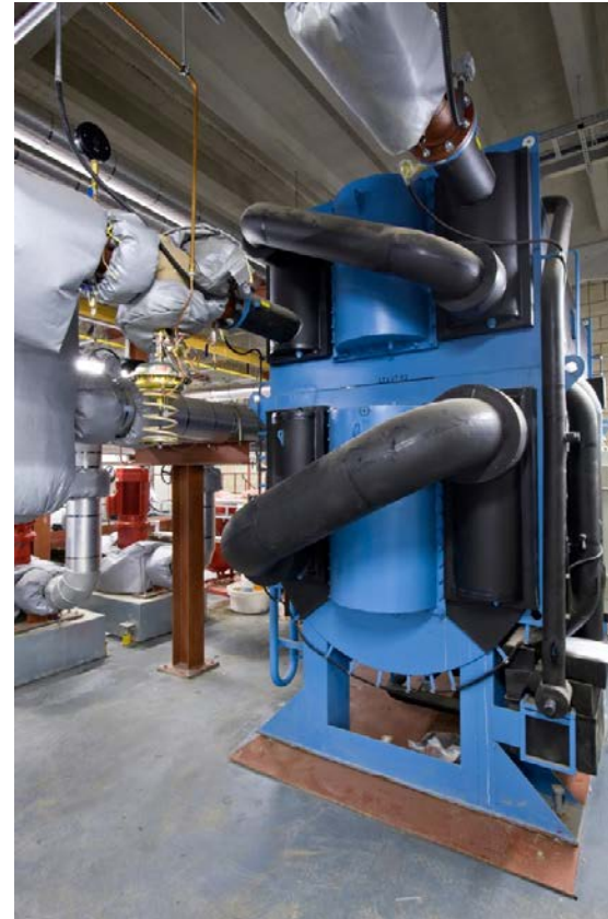
Two-Stage Indirect-Fired (Higher COP than single-stage) SIZE: up to 3,000 tons
