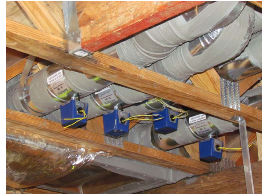
Installed Motorized Dampers (Blue control boxes)
