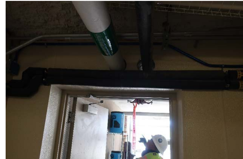
Pipe under pressure test.
