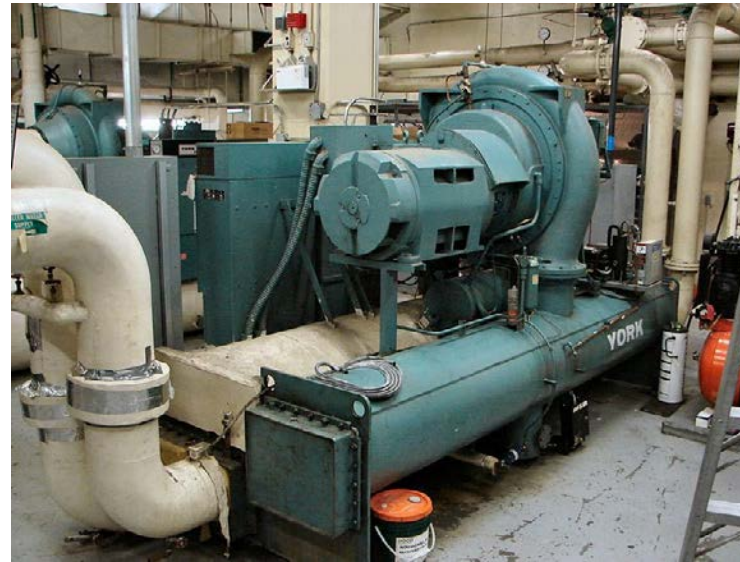
Water-Cooled Chiller with R-134A centrifugal compressor SIZE: up to 8,000 tons
