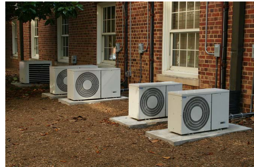
Condensing units outside a building
