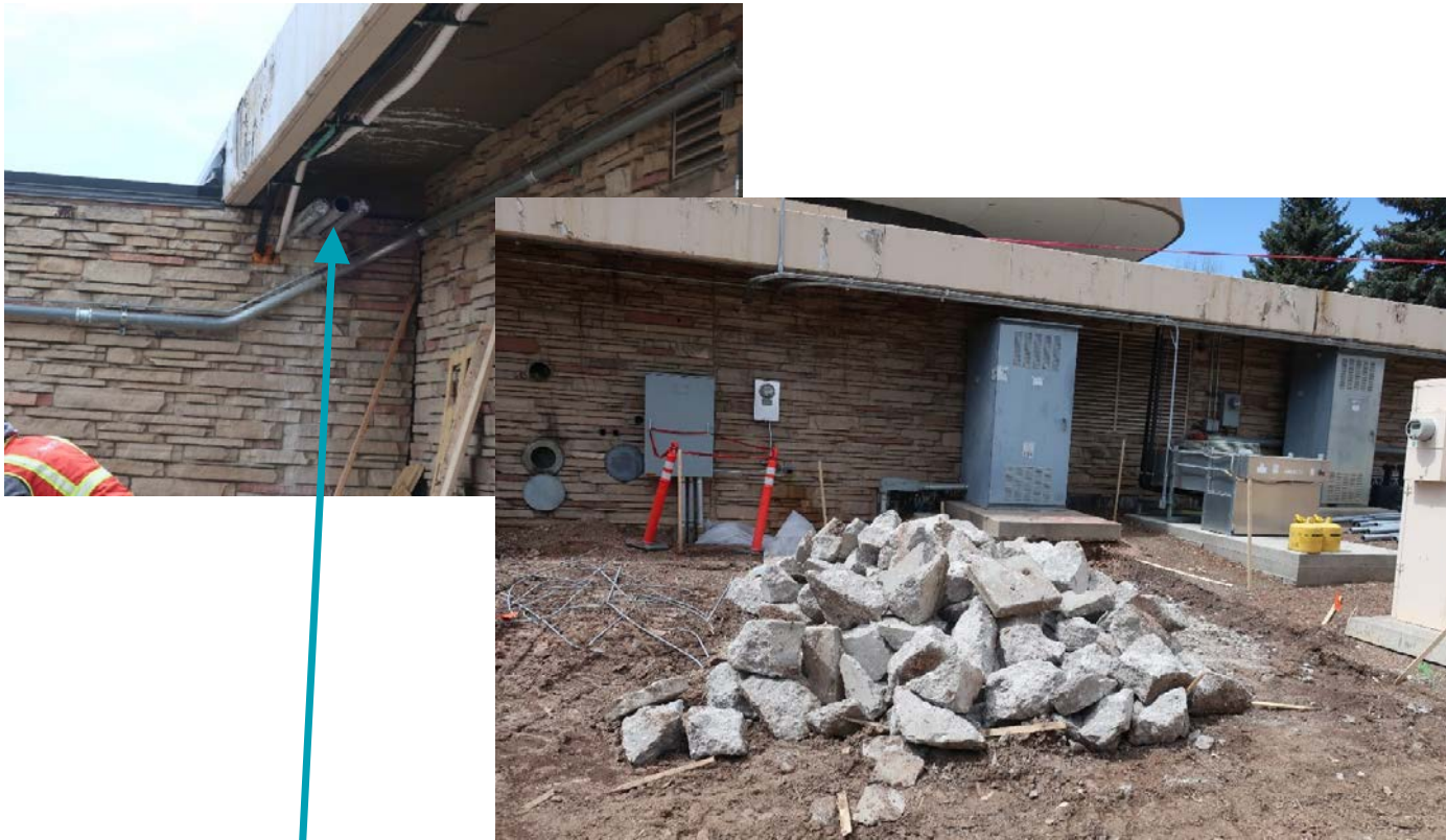
3- 4" new electrical conduits for new electrical room
