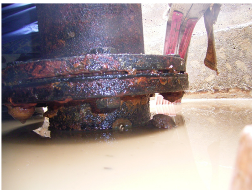
Photograph 2. Defect in air valve
