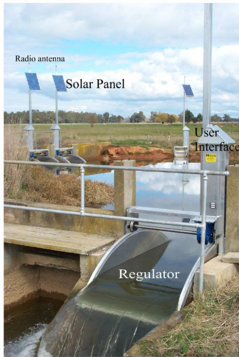
Figure 1. TCC™ hardware in Victoria, Australia
