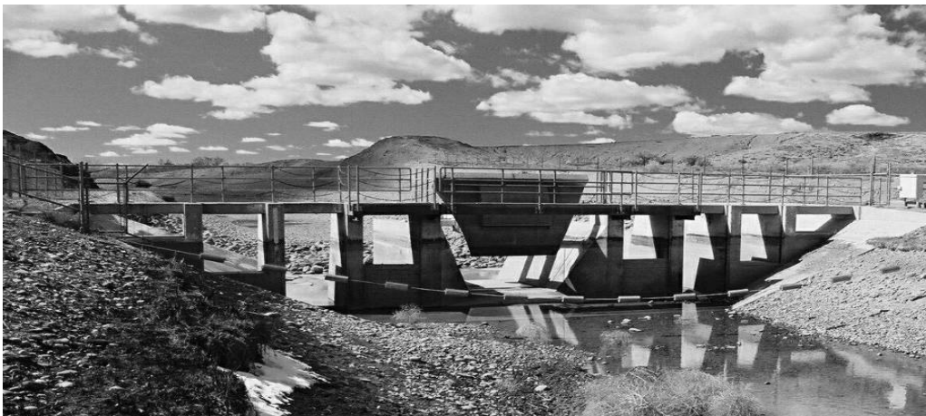
Figure 4. Amil Gate / Stop Log Structure
