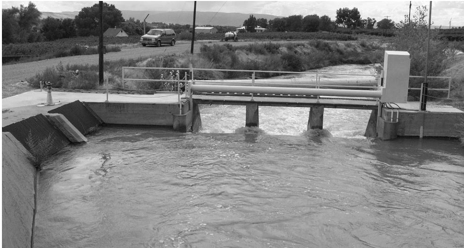
Figure 3. Gate Installed in Modified Stop Log Structure
