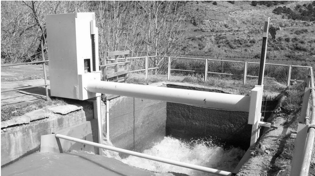
Figure 6. Siphon Inlet Flow Control
