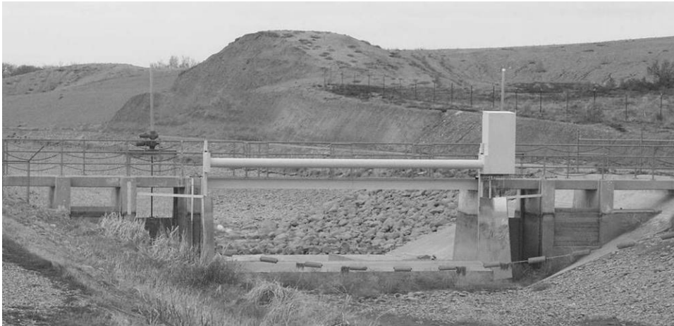
Figure 5. Langemann Gate Installed in Existing Structure
