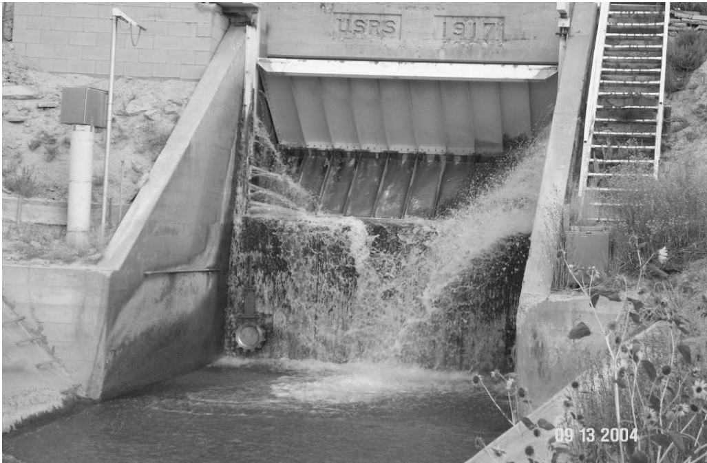
Figure 8. Highline Lake, Side-Channel Spillway
