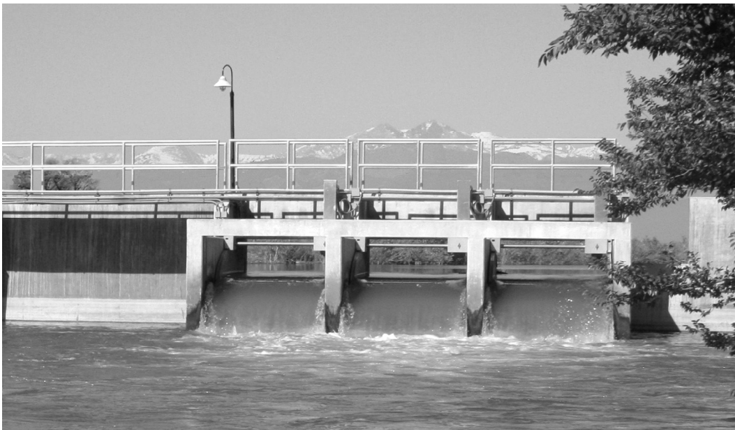
Figure 2. Rubicon Gates in Operation at Windsor Outlet
