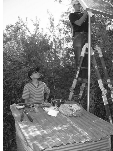
Figure 2. Installing a radio antenna and solar panel next to a shelter at a Parshall flume.
