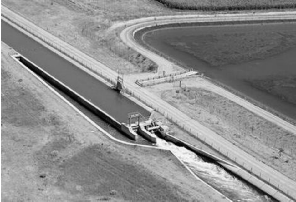
Figure 2. Paramo Bajo canal-Constant upstream/downstream water level gate combined with a reservoir.
