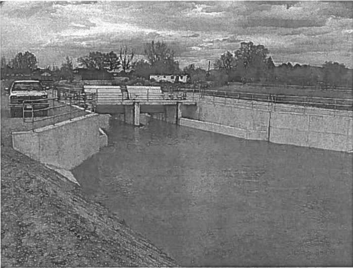
Figure 4. Typical Installation of Automatic Radial Gates and Long Crested Weirs
