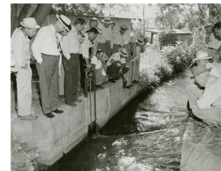
Viewing vortex tube sand trap in Jackson Ditch at Bellvue Hydraulic Lab, 1948. Photo from the Irrigation Research Papers, Water Resources Archive at Morgan Library.
