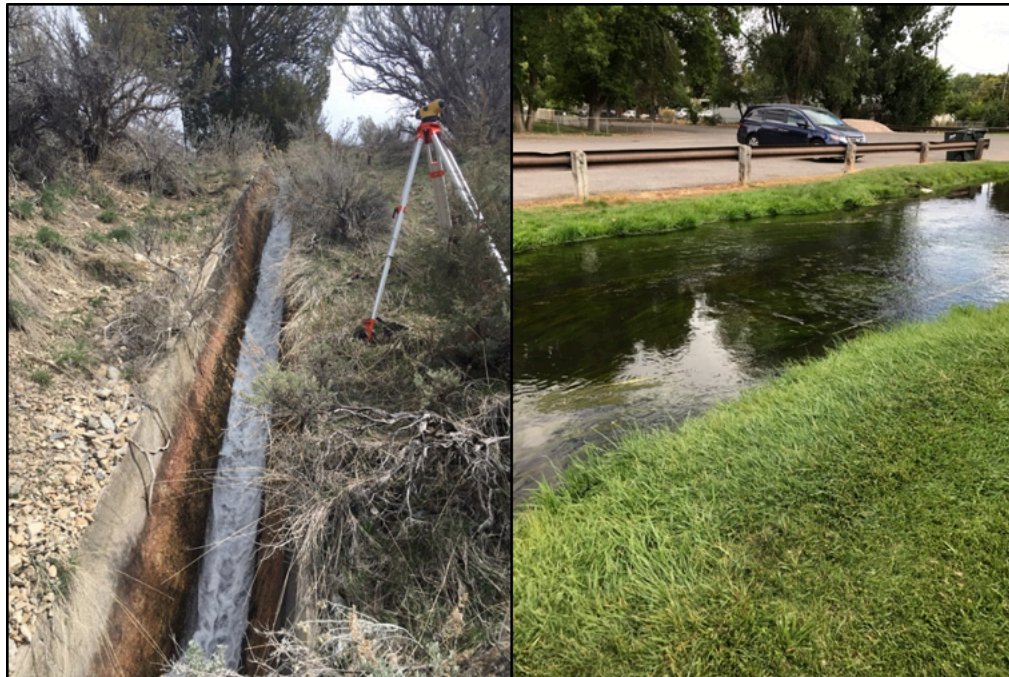
Fig. 4. Many canals in Utah were constructed along very steep slopes. In the left-hand photo, the Mt. Nebo Canal (Site UC2, see Table 4a) descends along a slope S = 0.3669 . In the lower part of the canal wall, the concrete finish has been stripped away to expose the rough aggregate underneath. In the right-hand photo, the Lions Park Canal (Site UC11, see Table 4a) is an earthen canal with banks of grass and dense weeds, descending at a slope S = 0.0052 .
