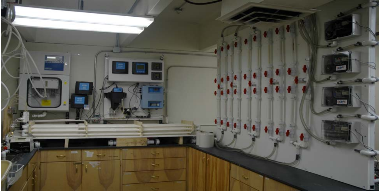
Figure 2-1 Bench-Scale Distribution System
