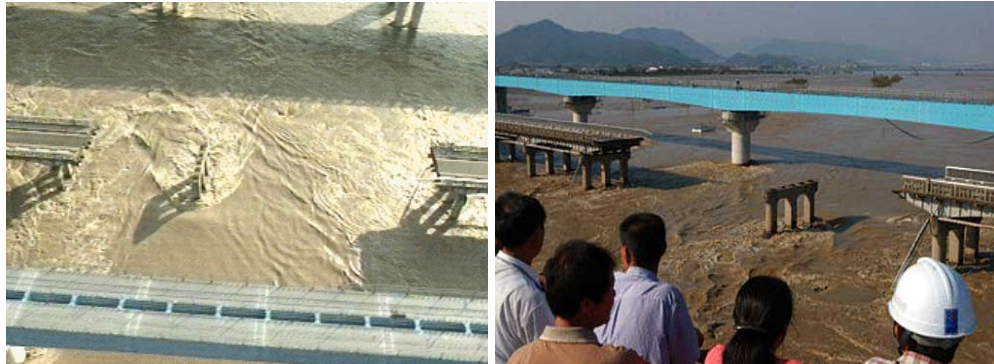
Figure 9. Gupo bridge failure after Typhoon Maemi [Yonhap]
